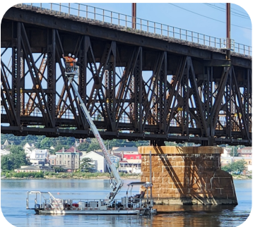
Maintenance on the NEC
