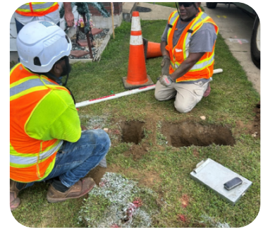
Identification of subsurface utilities
