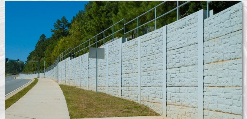
Typical Soldier Pile Wall
