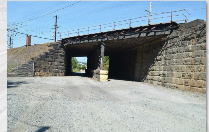
UG 59.52 - Access Road
