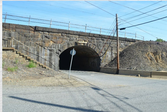
UG 59.39 - Access Road
