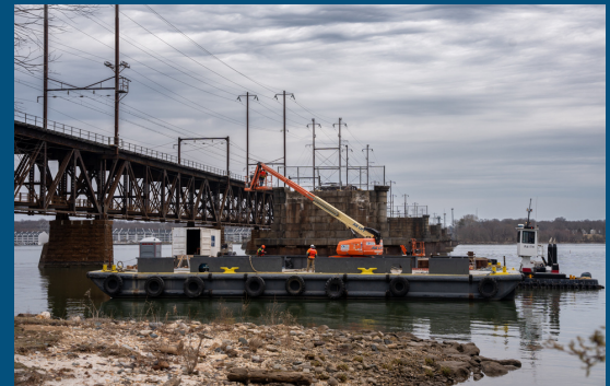
Installation of bird deterrent netting on the 1866 remnant piers.
