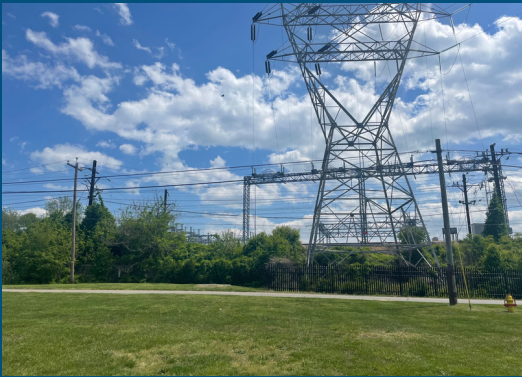
The existing transmission tower is located across from Rodgers Tavern in the Town of Perryville, Maryland. Property owners affected by the tower relocation project will be notified by BGE prior to the start of construction.
