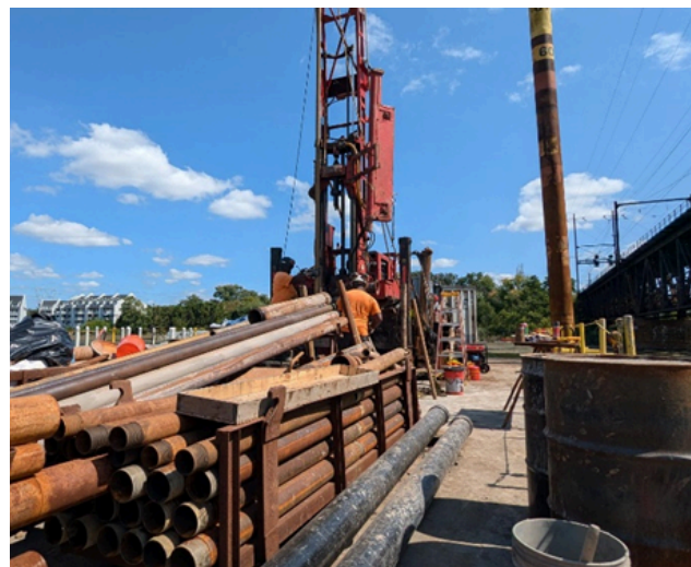
Proof borings being completed near the shoreline
