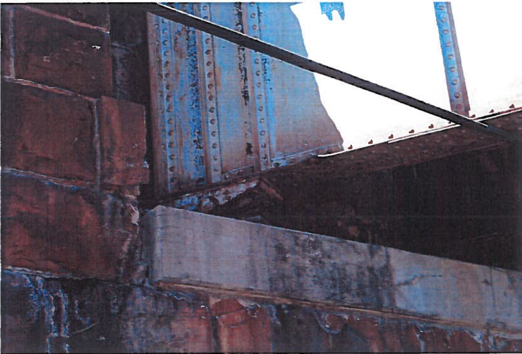
Abutment chop-out & capping at Juniata Street
