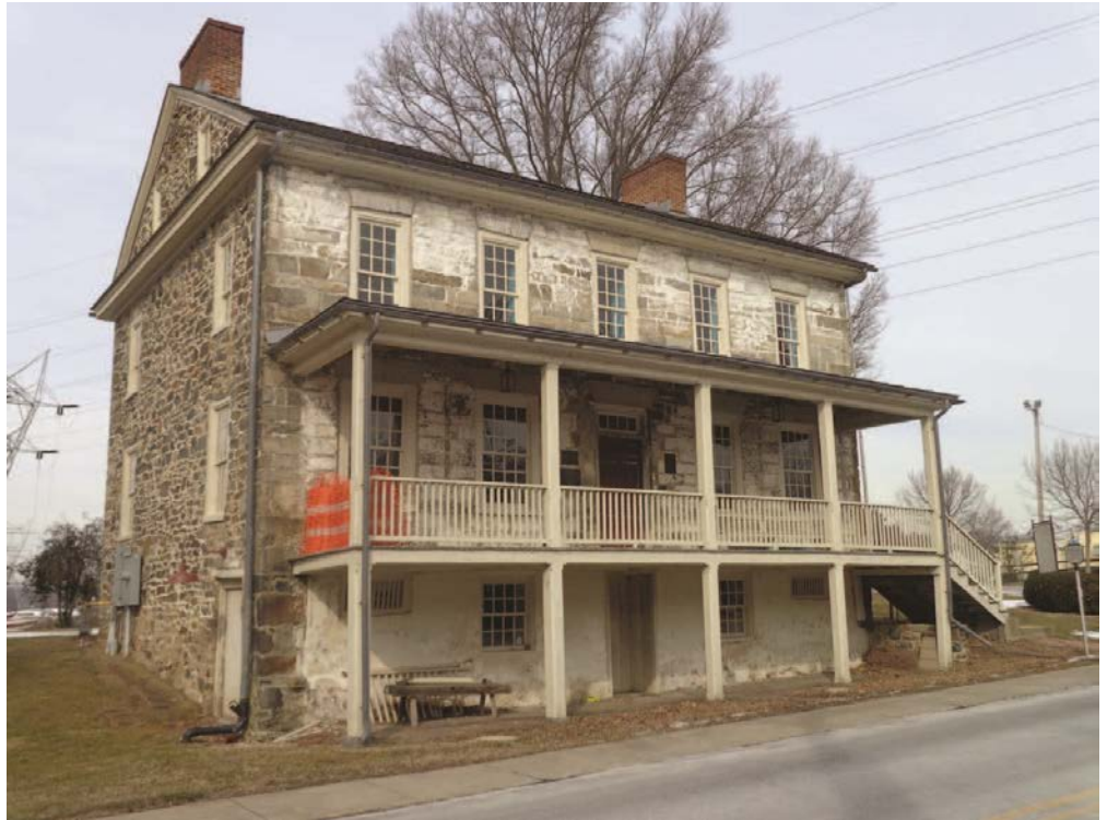
Rodgers Tavern: View of the front façade; looking north. 17
