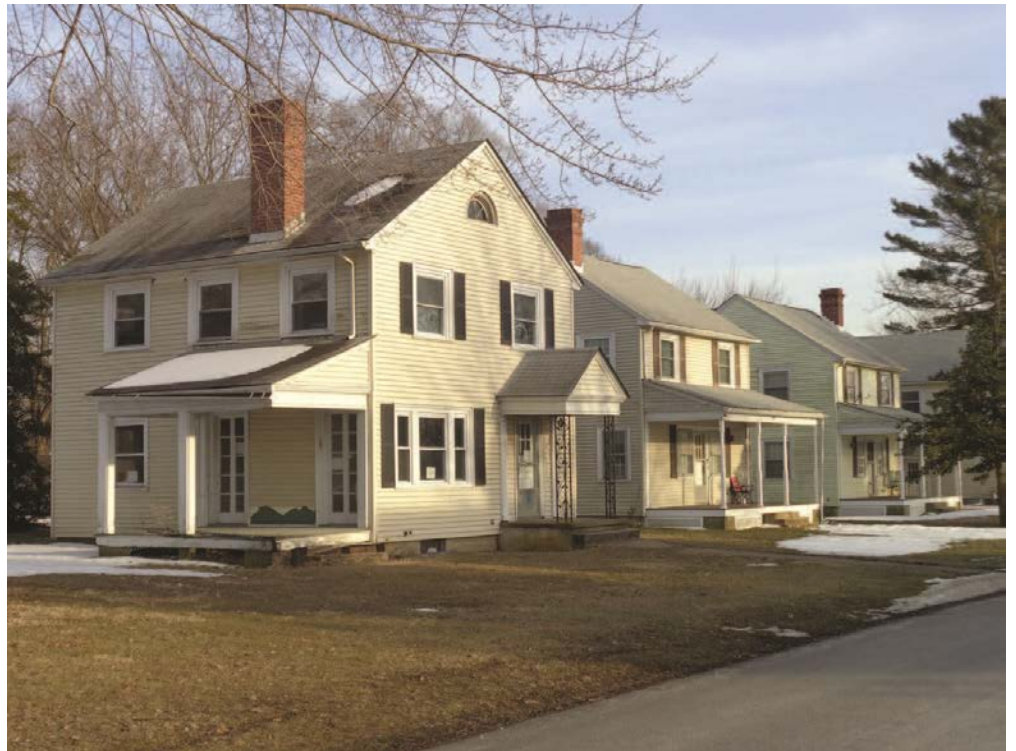
Perry Point Veterans Administration Medical Center: view of residences along Avenue D from 2nd Street; looking southeast. 28
