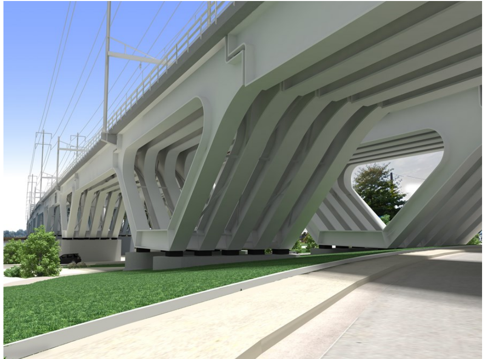
Rendering of the piers for the Delta frame approach; looking east from Havre de Grace. 36
