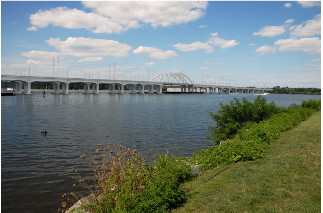
Rendering of a proposed replacement bridge with a girder approach and arch main span; 34 looking northeast from Havre de Grace.
