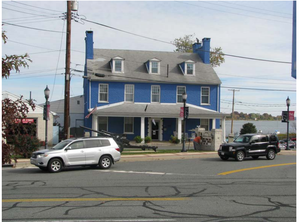
501 St. John Street: American Legion Building (former Lafayette Hotel); 1 looking east.
