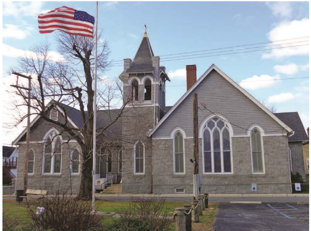
Perryville United Methodist Church: view of the east elevation; looking west. 30
