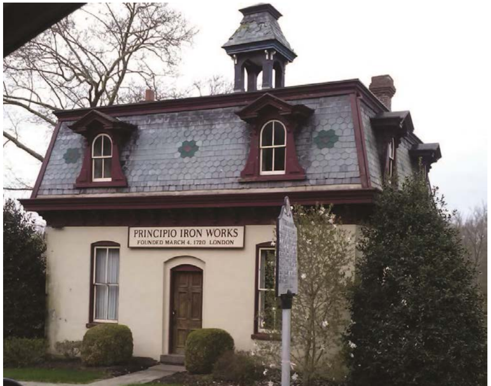
Principio Furnace Office Building; looking south. 18
