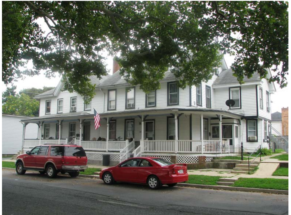
552 Warren Street: multi-family residential structure; looking southeast. 3
