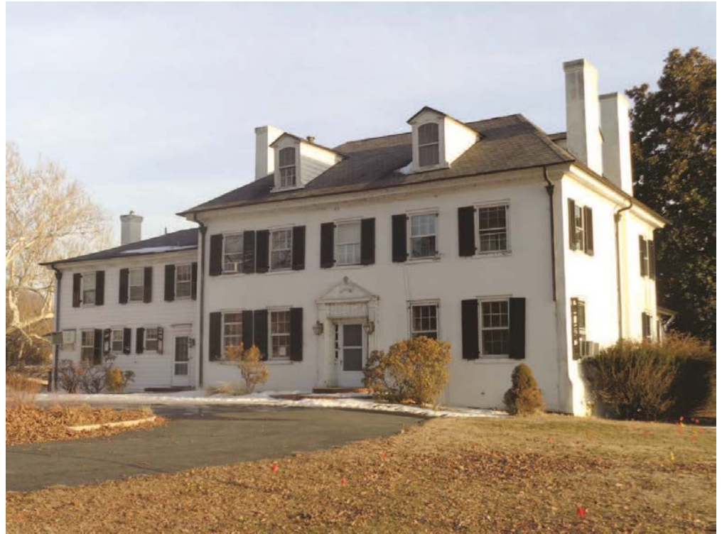
Perry Point Mansion House: view of the north façade; 19 looking south.
