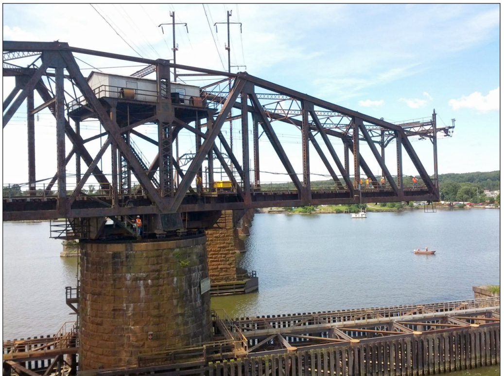
Opening swing span to accommodate marine traffic 2
