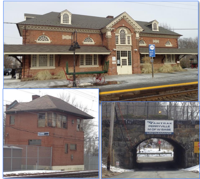
Perryville Station complex—Perryville Station, Perry Interlocking Tower, stone-arch bridge
