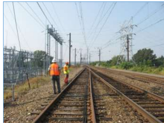
The Northeast Corridor merges from four tracks to two tracks (heading south from Perryville to Havre de Grace).
