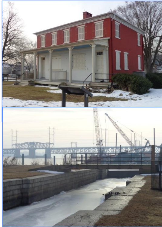
Southern Terminus, Susquehanna and Tidewater Canal - South Lock #1 and Toll House
