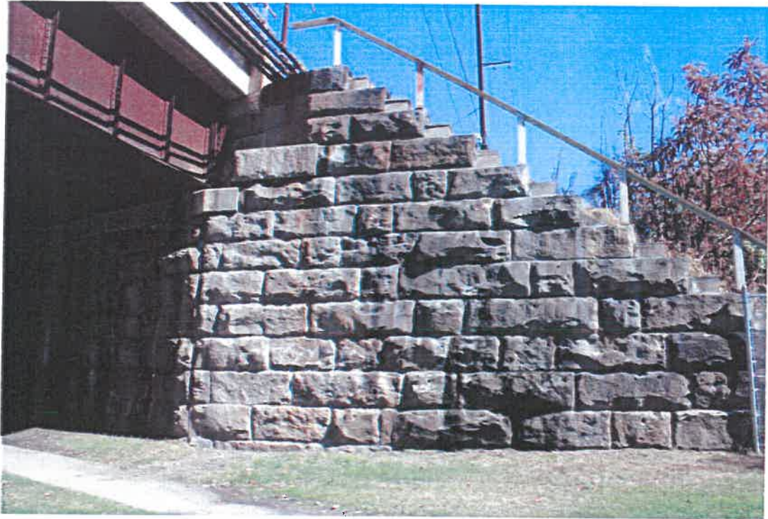
Chop-down & capping at Stokes Street abutment
