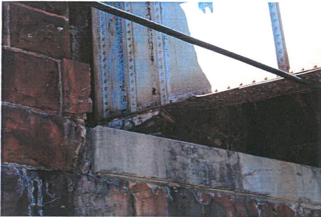
Abutment chop-out & capping at Juniata Street
