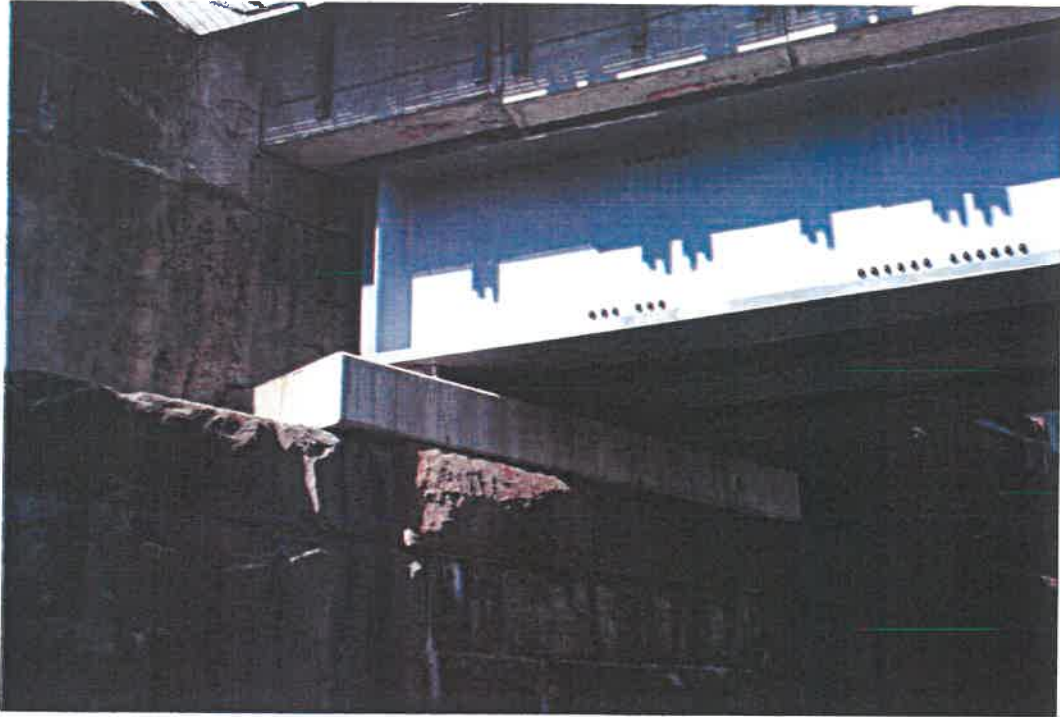
Concrete capping & chop-out at Adams Street
