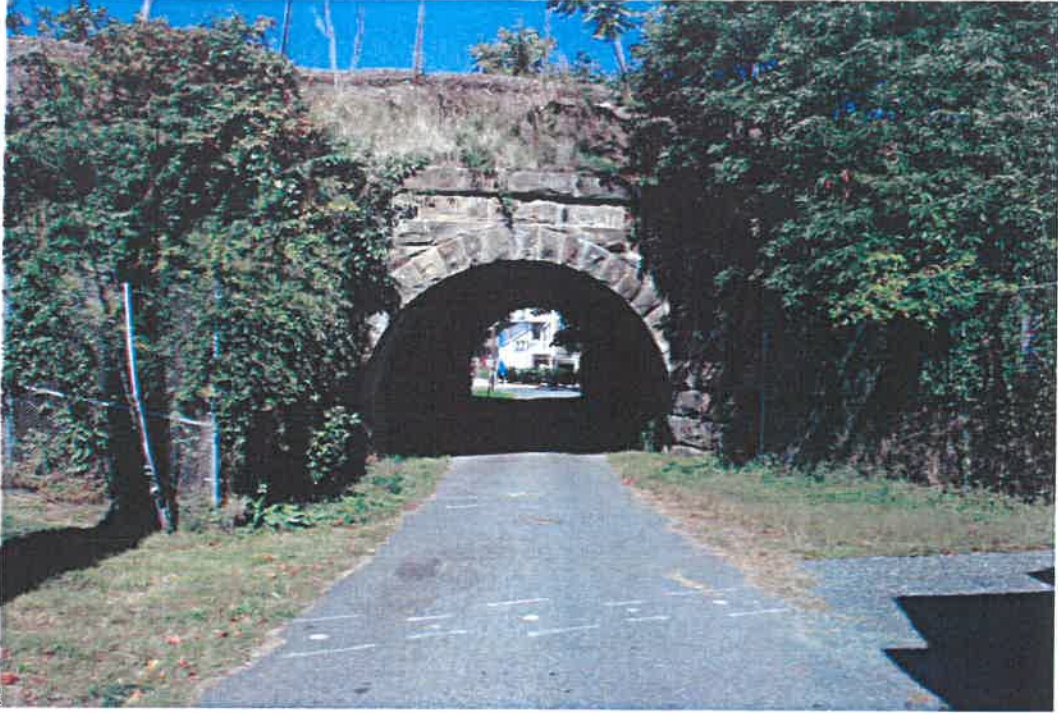
Freedom Lane overpass, south end
