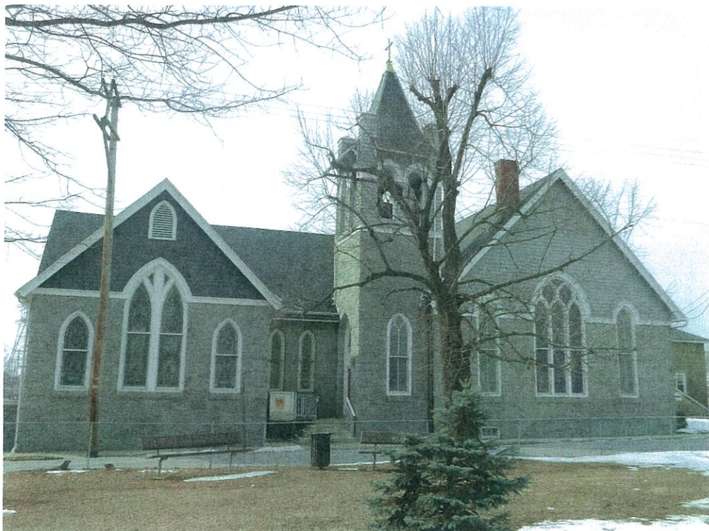
Figure 2: Perryville Methodist Church
