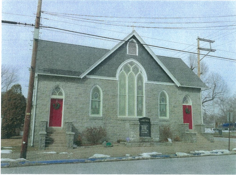
Figure 3: Perryville Methodist Church
