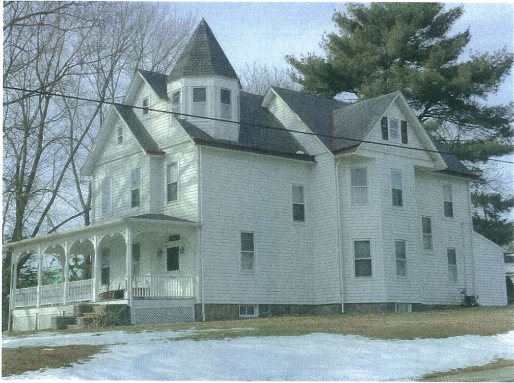
Figure 11: House at the corner of Broad Street and Cecil Avenue
