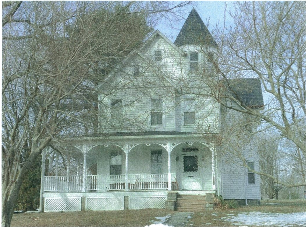
Figure 10: House at the corner of Broad Street and Cecil Avenue
