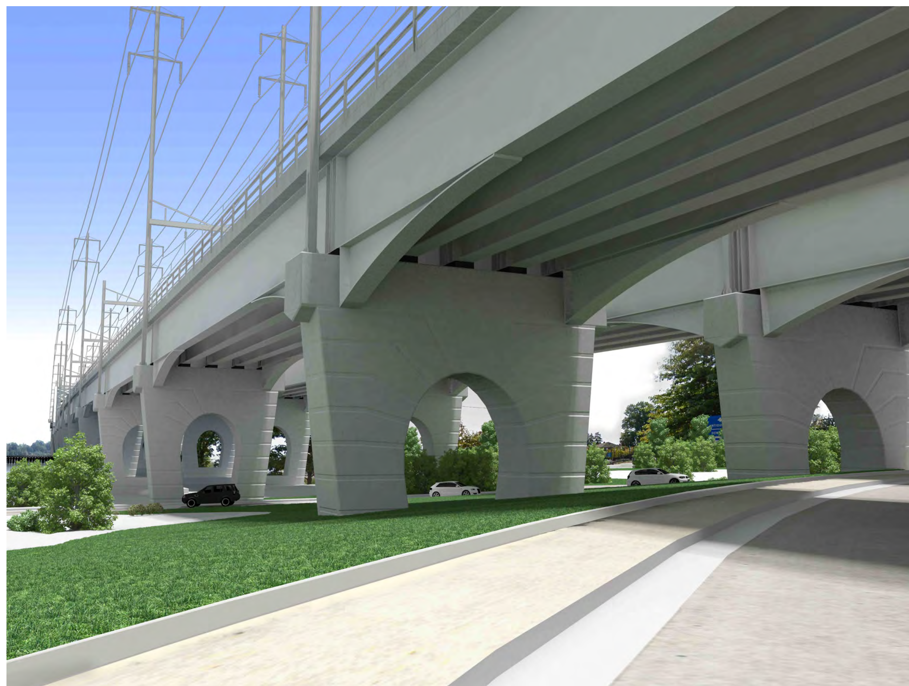
Key Hole Pier Design
