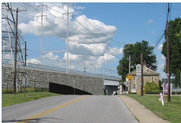
Retaining Wall with Haunched Girder Design
