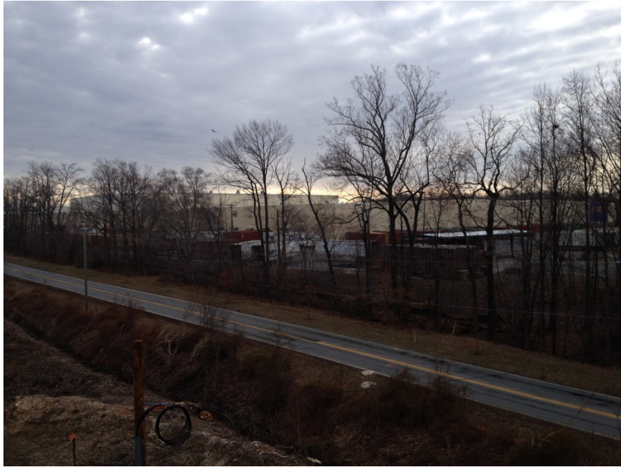
The IKEA site (former Firestone Plant) and Amtrak MOW access road, view to the southeast from Firestone Road bridge.
