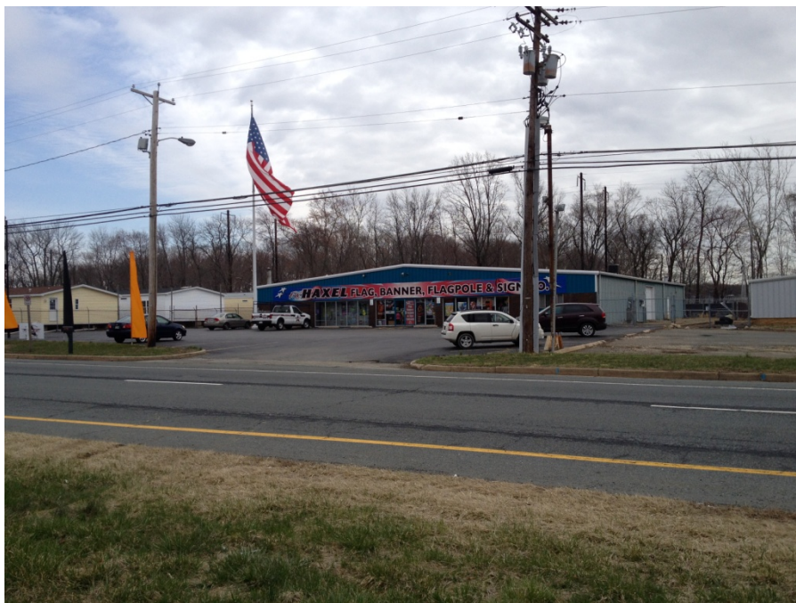
F.W. Haxel Co. site, view to the southeast from Pulaski Highway.
