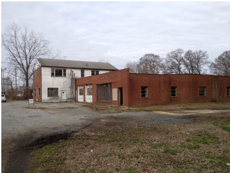
Perryville Oil Company site, view to the northwest from Otsego Street.
