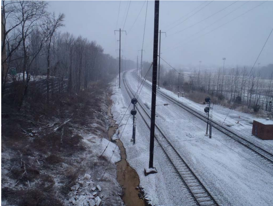
Photograph 5: General view of disturbed Amtrak ROW east of Lewis Lane, facing northeast.
