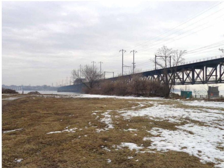
Photo 71: View looking northeast at the Jean S. Roberts Memorial Park where there will be a small taking of property.
