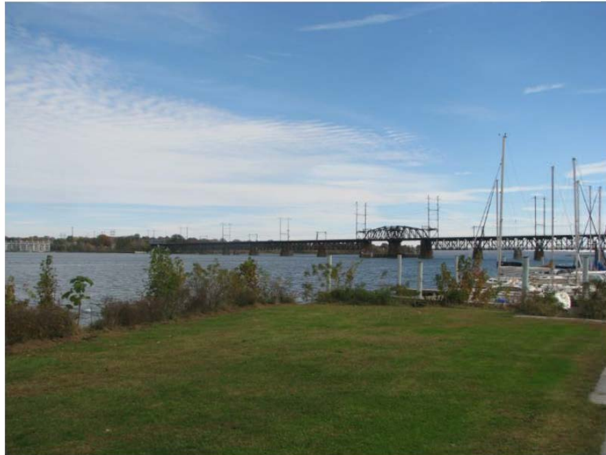
Photo 2: View looking southeast towards the Susquehanna River Rail Bridge from the Southern Terminus, Susquehanna and Tidewater Canal.
