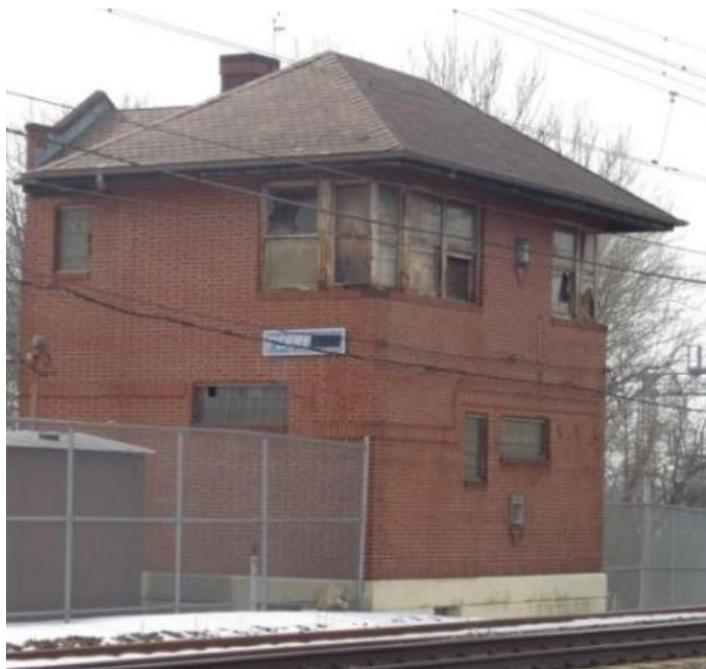
Photo 37: View looking southwest at the Perry Interlocking Tower.
