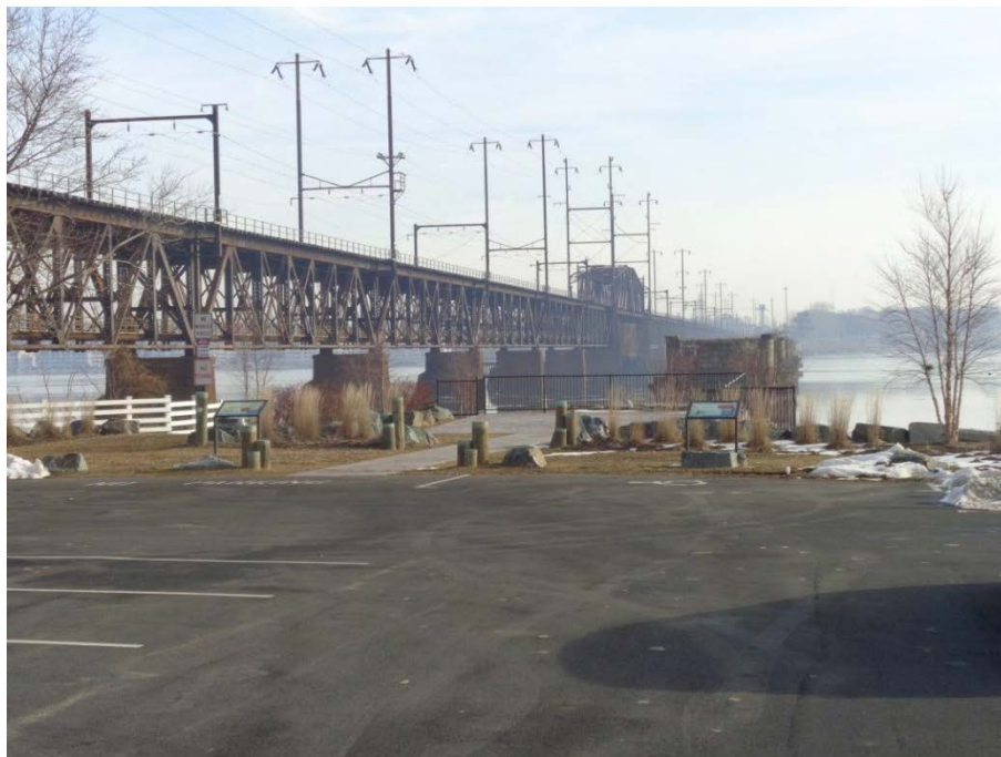
Photograph 1: Representative view of Havre de Grace waterfront near the existing Susquehanna River Bridge structure, looking east.
