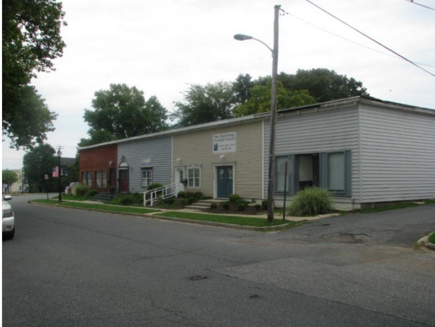
Photo 11: View looking east along Warren Street at a nineteenth century commercial structure that have suffered from a loss of architectural integrity.
