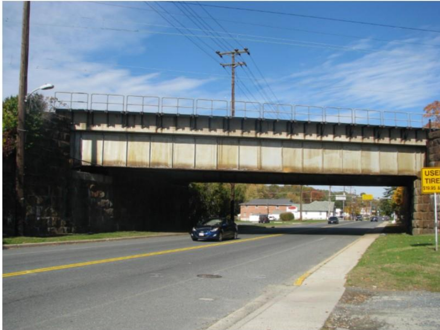
Photo 63: View looking northwest at the railroad east side of North Juniata Street Undergrade Bridge (MP 60.77), which will be altered via construction of a new concrete abutment.
