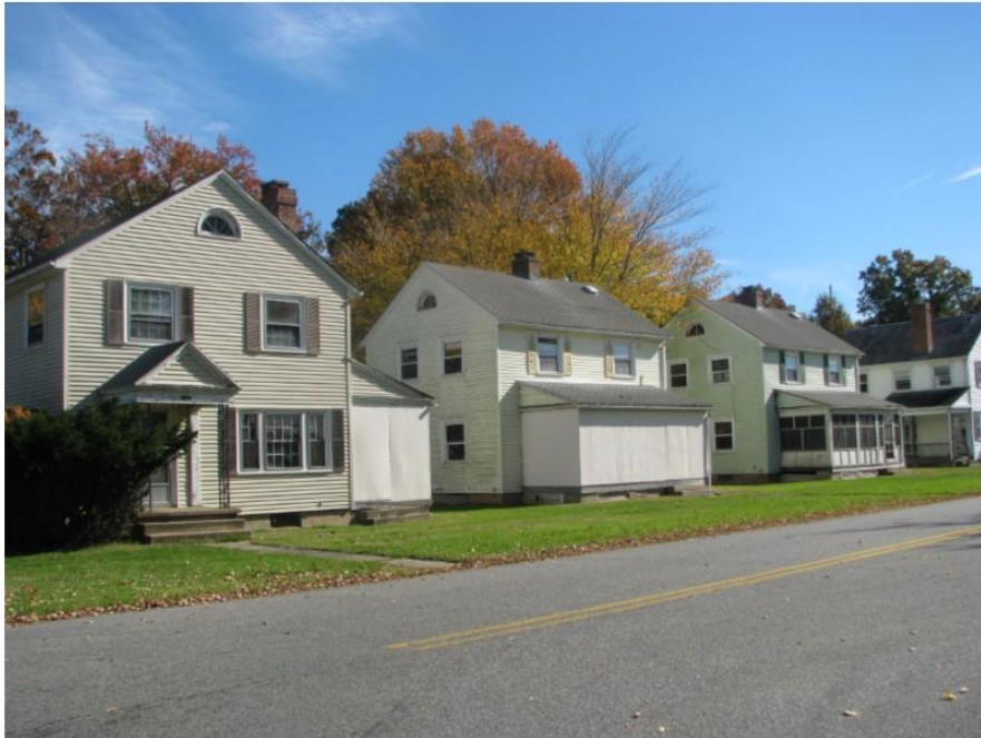
Photo 40: View looking east at representative houses along Avenue D within the Perry Point Veterans Administration Medical Center Historic District.
