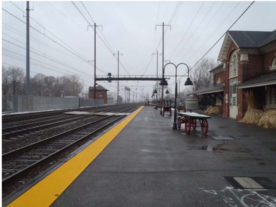
Photograph 10: General view of Perryville Station, facing west.
