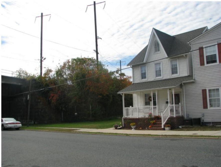
Photo 68: View looking southwest at the mid-nineteenth century house at 518 N. Stokes Street in relation to the railroad tracks. The setting of this house will be altered by the proposed widening that will bring the tracks 26-28 feet closer to it.
