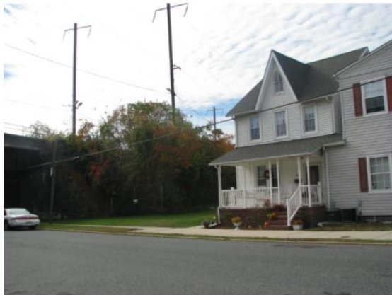
Photo 76: View looking southwest at 518 N. Stokes Street.
