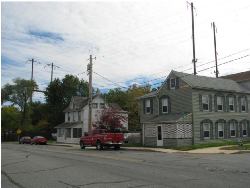
Photo 22: View looking southeast at two vernacular mid-nineteenth century houses at the southeast corner of Otsego Street and N. Stokes Street.
