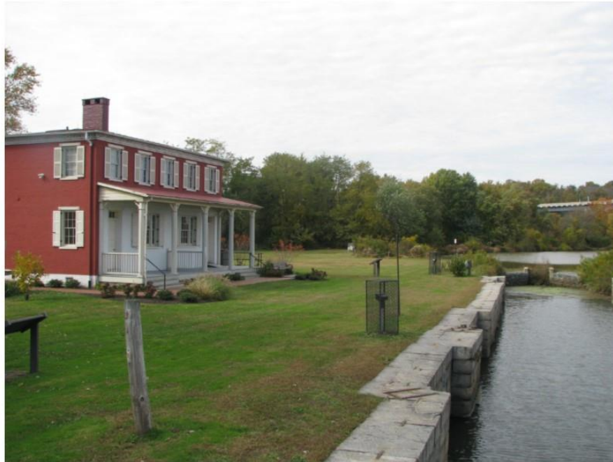
Photo 32: View looking north at the Southern Terminus, Susquehanna and Tidewater Canal- South Lock #1 and Toll House.
