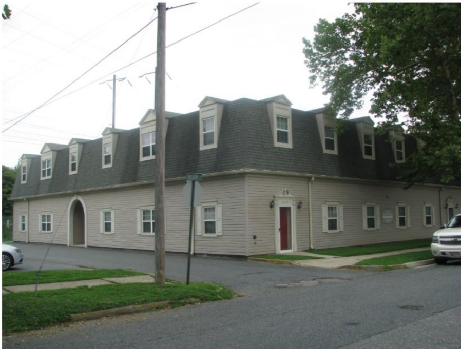
Photo 12: View looking northeast at a large modern one-story residential structure at 515 Warren Street.
