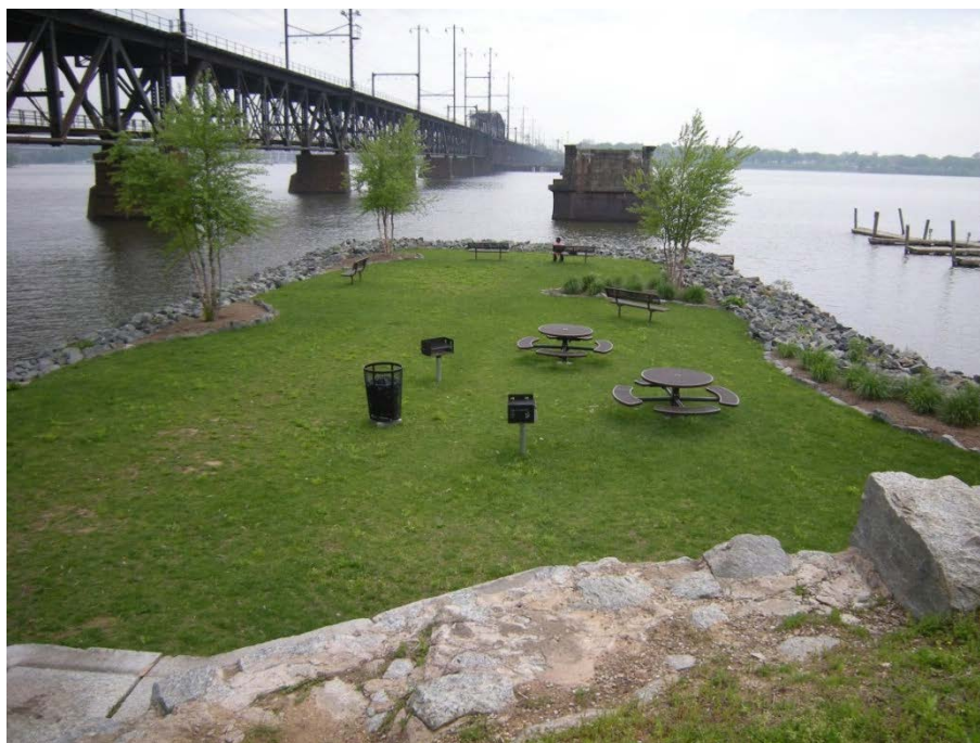
Photograph 23: View of David Craig Park (Study Area 3), facing east-northeast. Note PW&B abutment in foreground.
