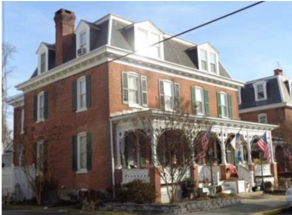
Photo 3: Representative mid-nineteenth century residential structure within the Havre de Grace Historic District.
