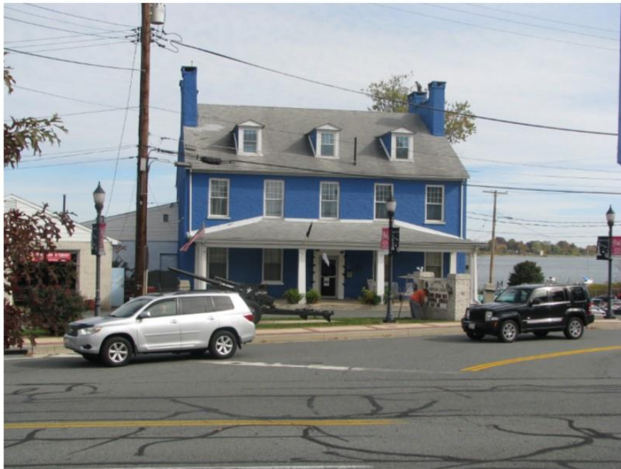
Photo 8: View looking east at the American Legion Building, the former Lafayette Hotel, 501 St. John Street, Havre de Grace.
