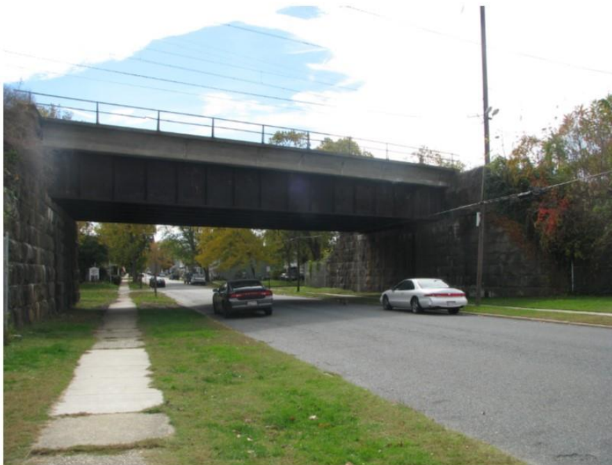
Photo 58: View looking south at the railroad west side of North Stokes Street Undergrade Bridge (MP 60.56), which will be altered via removing a portion of the existing stone masonry abutment and building new concrete abutment.
