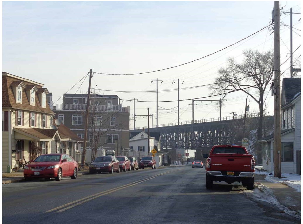
View looking east from Otsego and North Stokes Streets towards the Susquehanna River Rail Bridge approach span. 10
