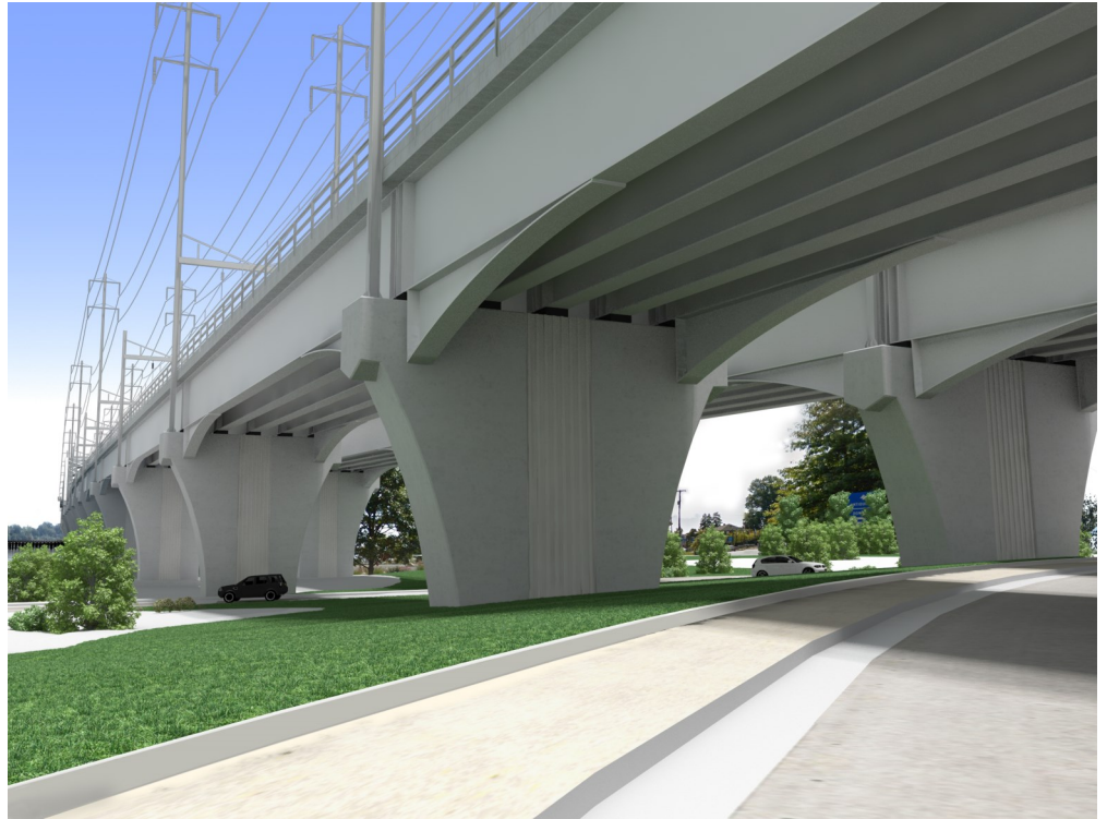
Rendering of possible Fluted Piers to be used with the Girder Approach. 35
