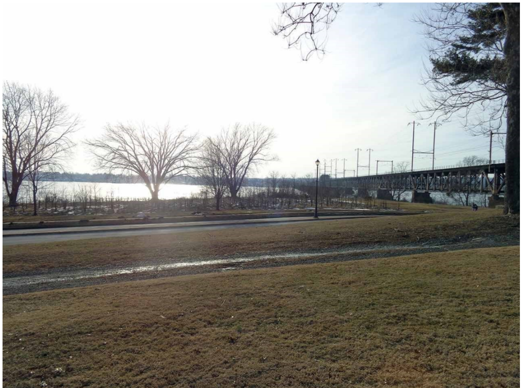
View looking northwest towards the Susquehanna River Rail Bridge and Susquehanna River from a walking path that follows the shoreline of the Perry Point VA Medical Center property. 14
