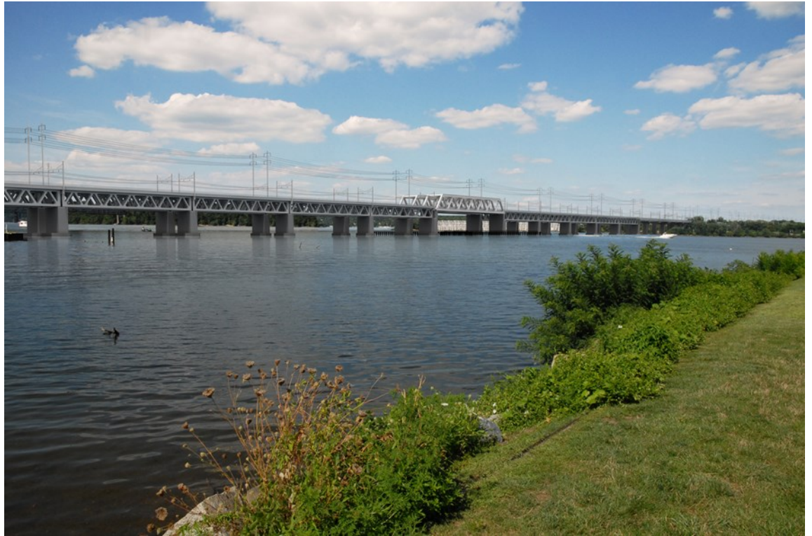
Rendering of a proposed replacement bridge with a Truss Approach and a Truss Main Span. 31
