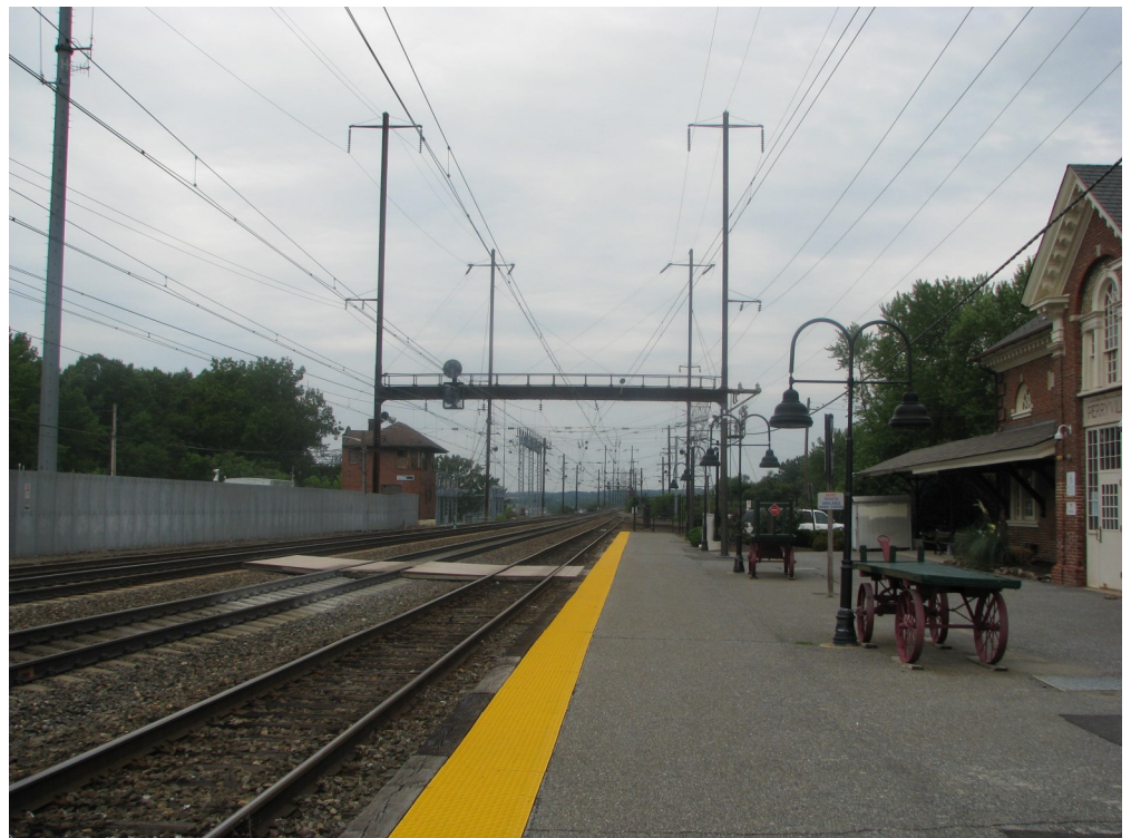
View looking southwest along the NEC at the Perryville Railroad Station (right) and the Perry Interlocking Tower (left). 16
