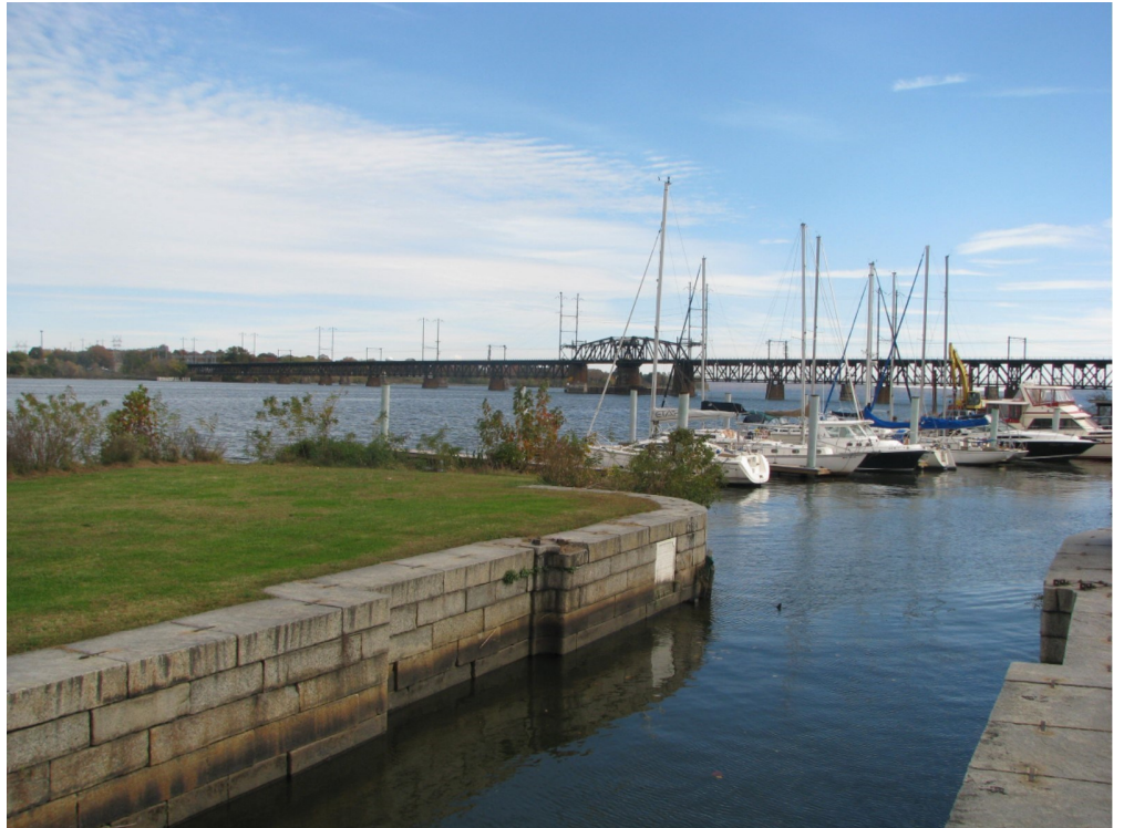
View looking south from the Southern Terminus, Susquehanna and Tidewater Canal - South Lock #1 and Toll House towards the Susquehanna River Rail Bridge in the distance. 12
