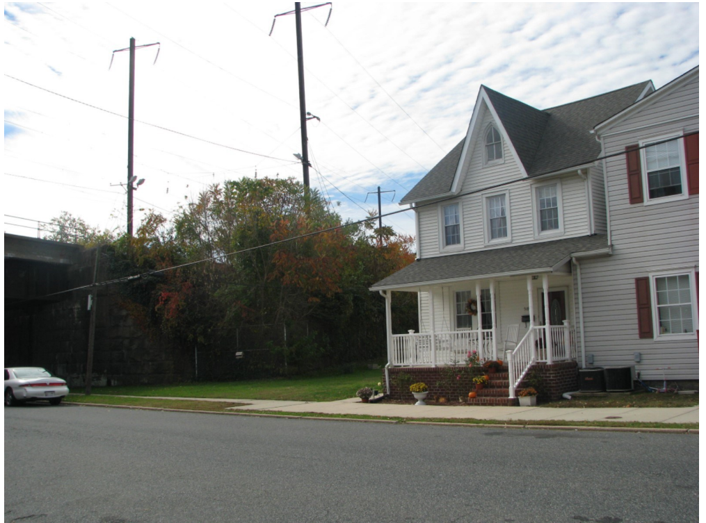
View looking southwest from North Stokes Street towards the NEC embankment. 11
