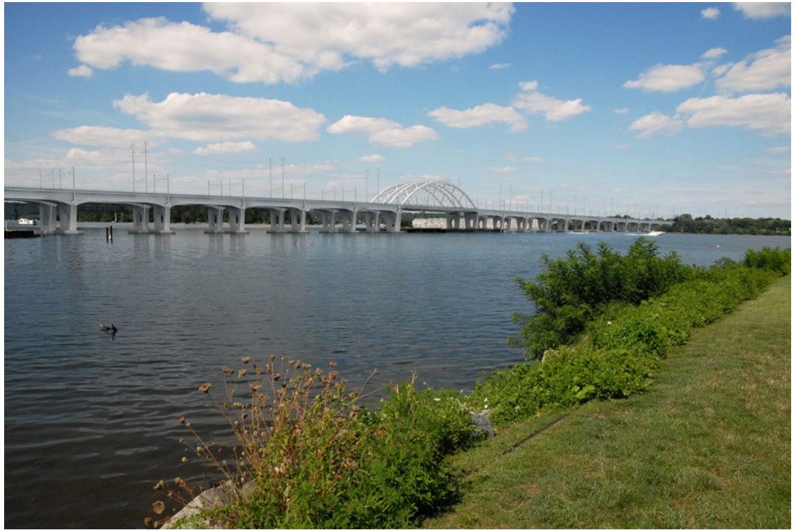
Rendering of a proposed replacement bridge with a Girder Approach and Arch Main Span. 29
