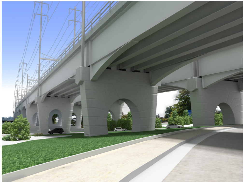
Rendering of possible Arched Piers to be used with the Girder Approach. 34
