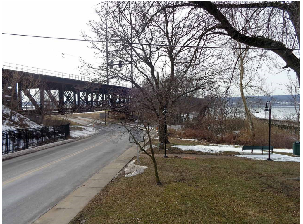
View looking southwest along Board Street towards the Susquehanna River Rail Bridge, abutment, and underpass in front of Rodgers Tavern. 25
