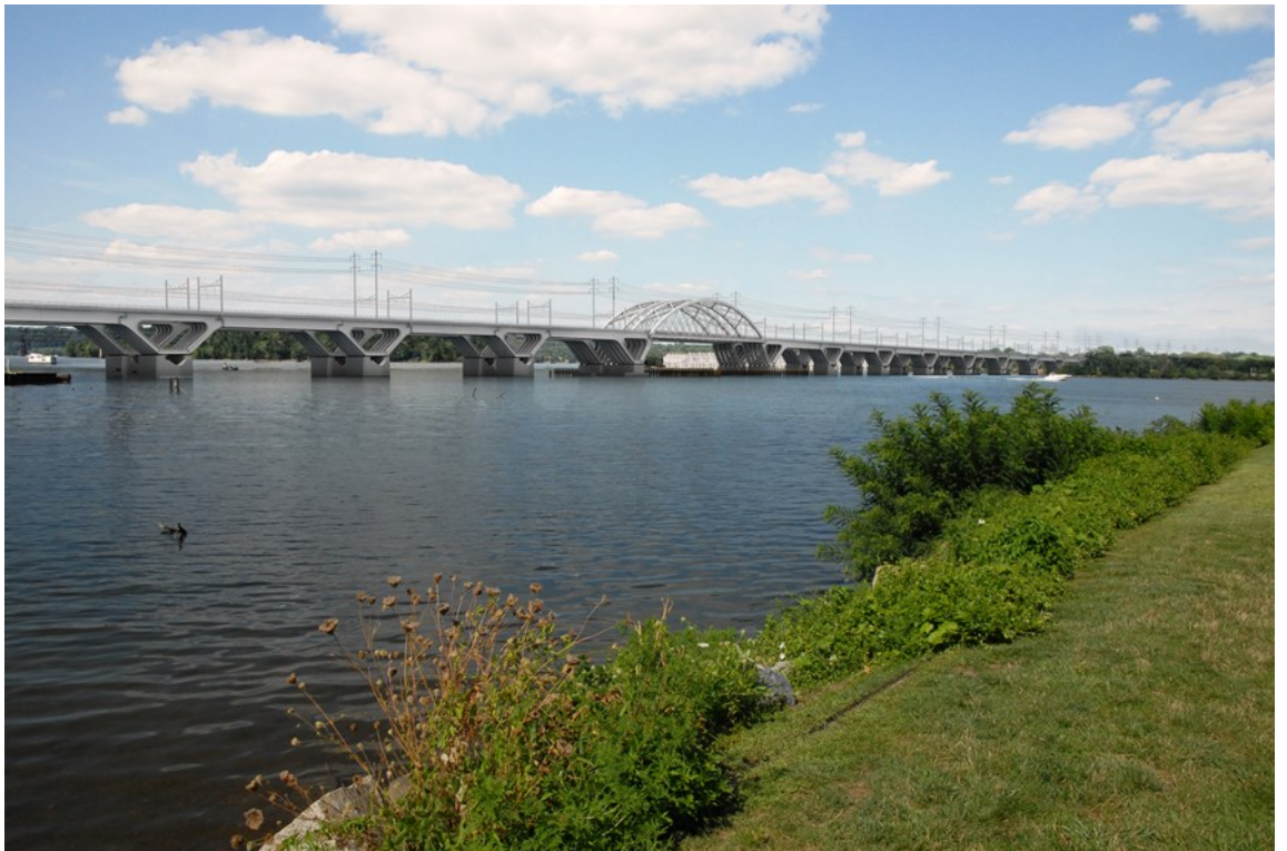
Rendering of a proposed replacement bridge with a Delta Frame Approach and Arch Main Span. 30
