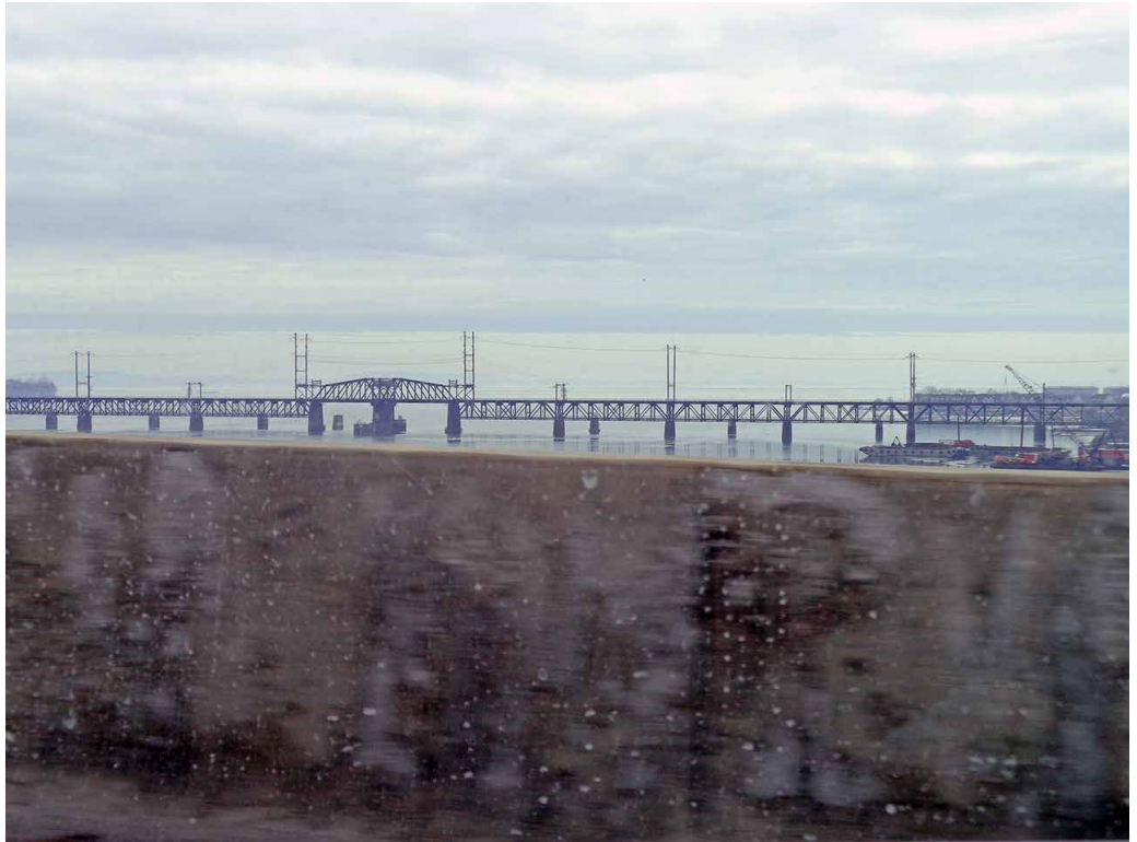
View looking south towards the Susquehanna River Rail Bridge from the 23 Thomas J. Hatem Memorial Bridge.
