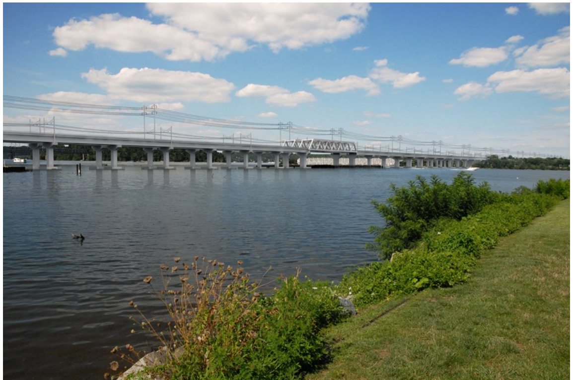
Rendering of a proposed replacement bridge with a Girder Approach and a Truss Main Span and a wall pier design. 32
