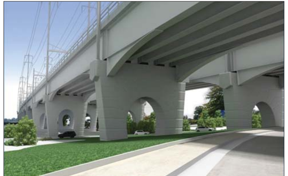
Key Hole Pier Design
