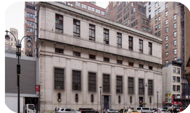
Interior renovation of Penn Station Service Building
