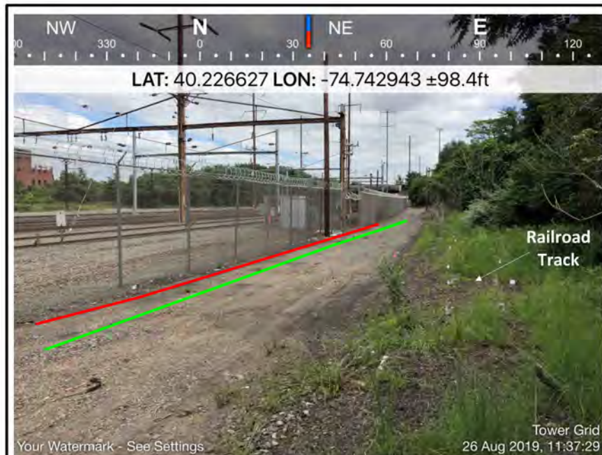
Photo 3: The photo shows the approximate location of the 5.5-foot diameter storm line next to the fence, an electric line, and an unknown line. The approximate photo location, direction the photo was taken, and the date and time of the photo is presented.
