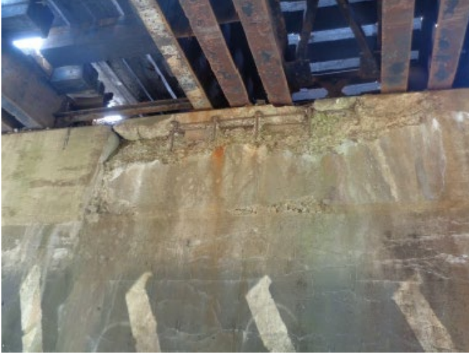
WEST ABUTMENT SPALLING UNDER BEARINGS
