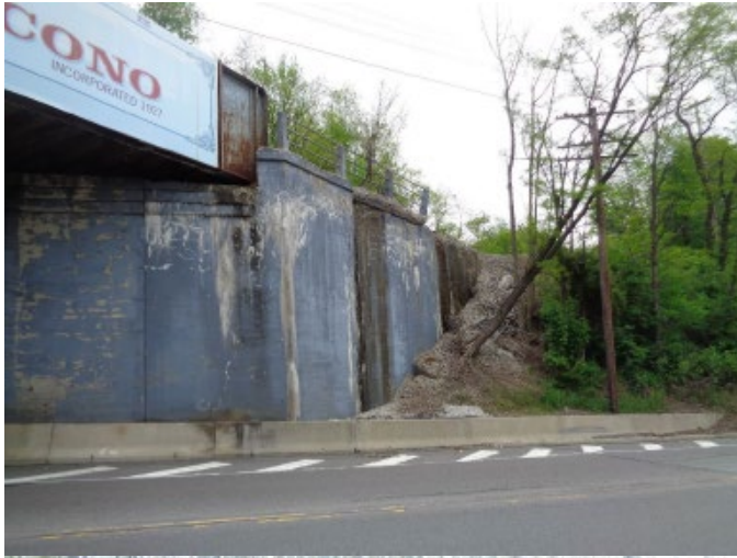
DETERIORATED SE WINGWALL
