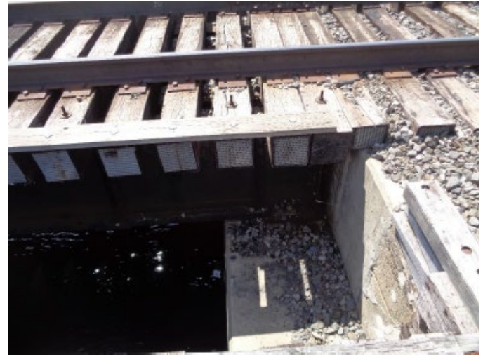
WEST ABUTMENT BRIDGE SEAT
