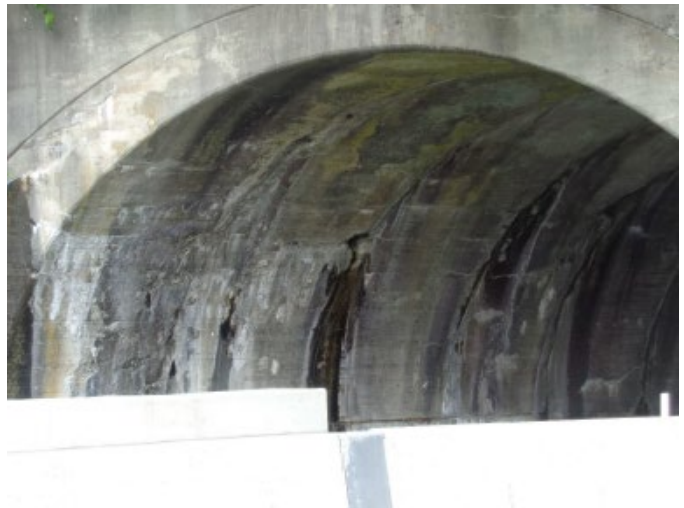
TYPICAL JOINT LEAKAGE
