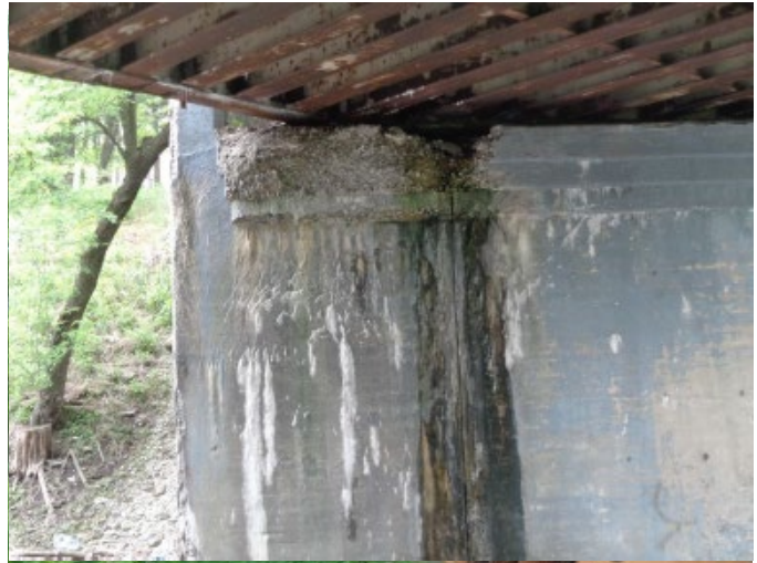
DETERIORATED BRIDGE SEAT ON EAST ABUTMENT
