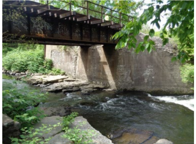
WEST ABUTMENT SPALLING
