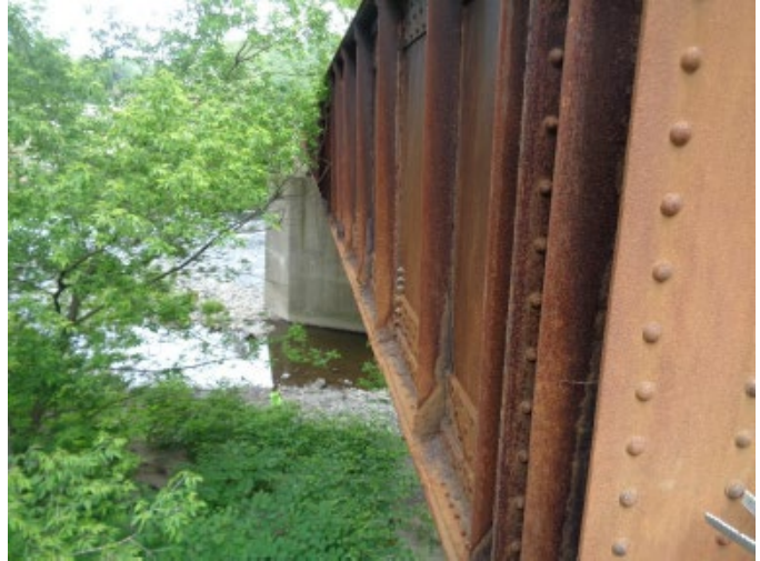
INTERMEDIATE STIFFENER CORROSION NORTH GIRDER
