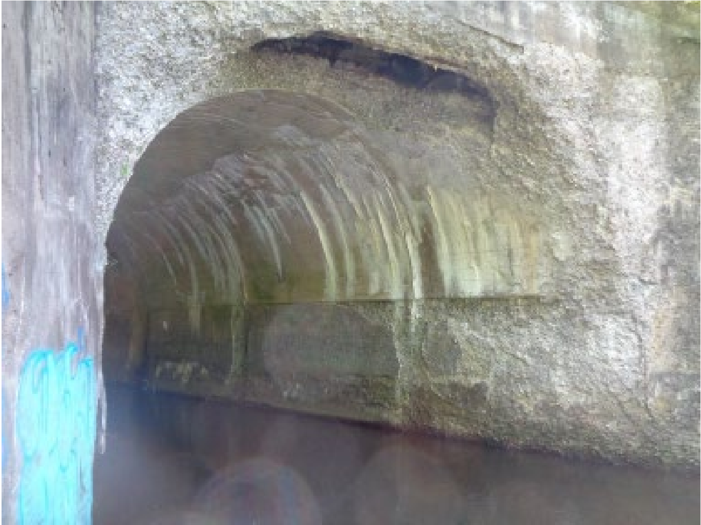
LARGE DEEP SPALL ON NORTH HEADWALL
