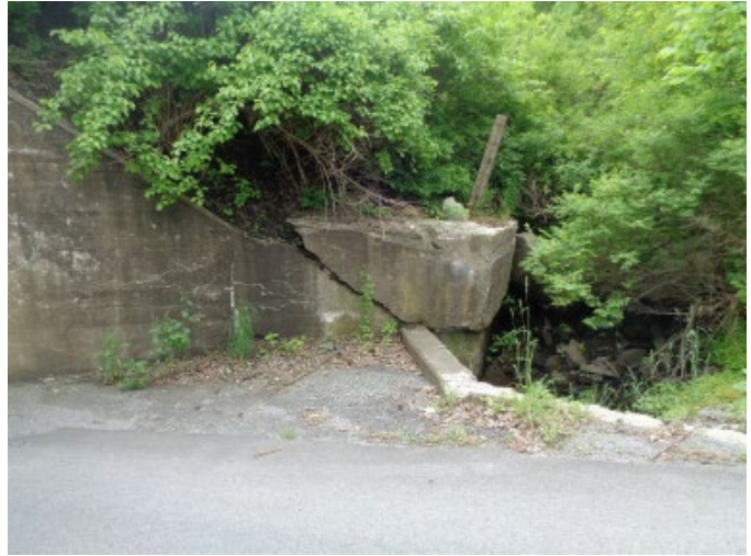
SE WINGWALL CRACKED & DISPLACED
