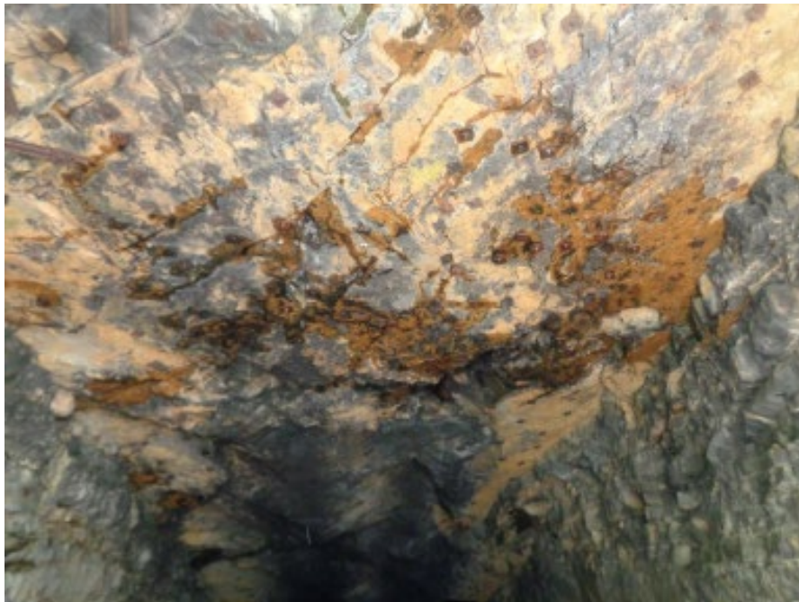
ROCK BOLTS IN THE CEILING AT WEST ENTRANCE NORTH BORE
