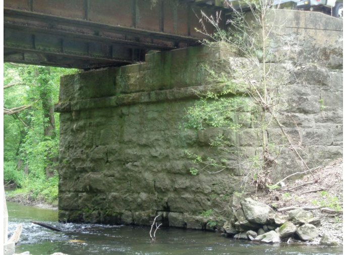
EAST ABUTMENT, SOME CRACKS
