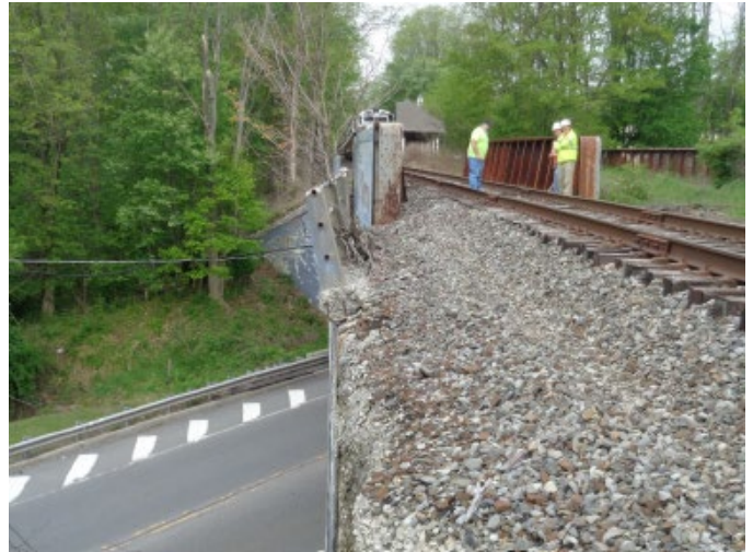
RAILING DETERIORATED ON SE SIDE
