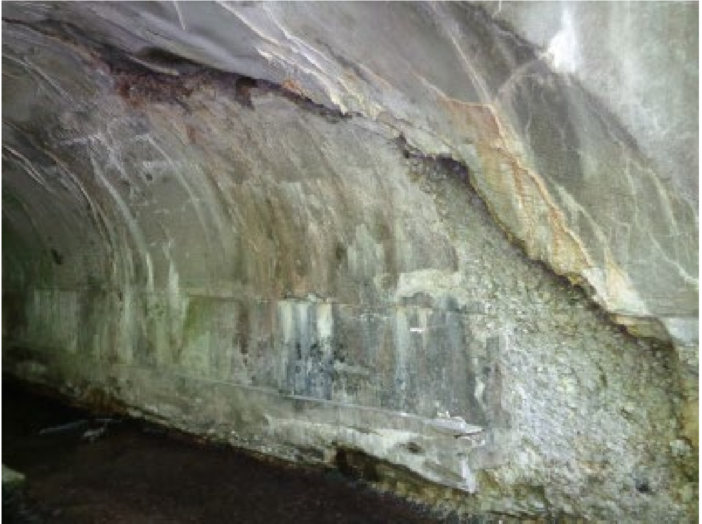
SPALLING IN WEST CULVERT WALL
