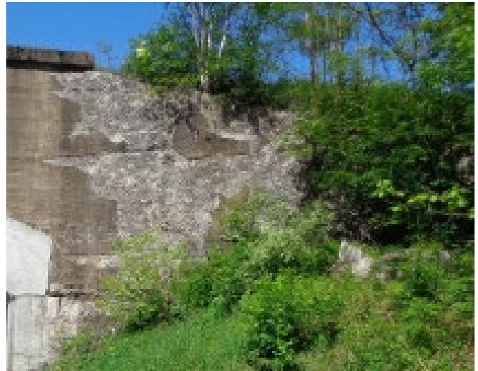
WINGWALL SPALL DETAIL LOOKING NORTH
