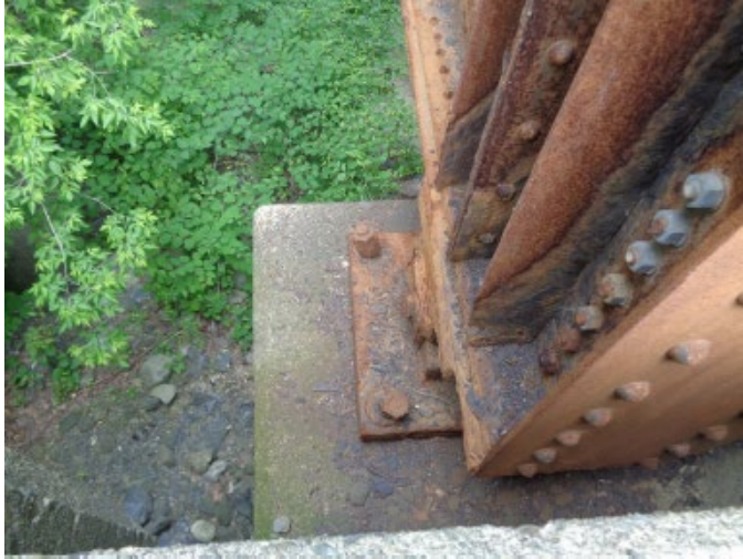
BEARING AT SE CORNER OF ABUTMENT
