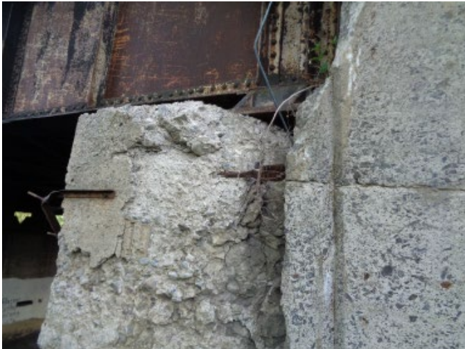
UNDERMINED BEARING NEAR BIKE PATH (SPAN 5)
