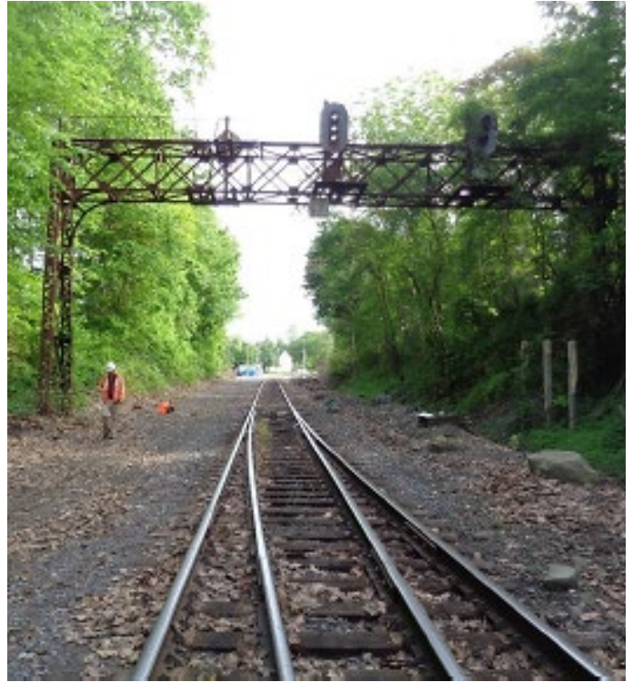
TYPICAL DL&W SIGNAL BRIDGE
