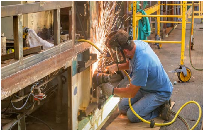
Skilled employees at heavy maintenance facilities in Indiana and Delaware rebuild and overhaul a wide variety of cars and locomotives.
