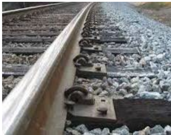
Figure 15 Woodings Rail Anchor (Left) & Wood Tie with e-Clip (Victor Plate)
