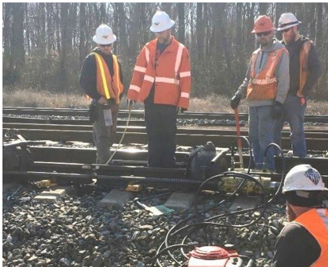
Figure 19 Re-adjusting Plug Rail Location
