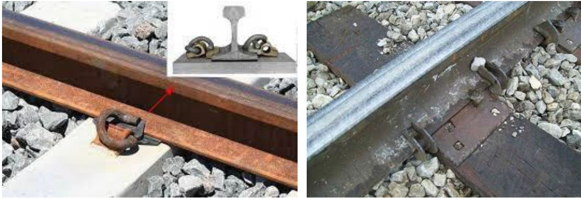
Figure 13 e-Clip on Concrete (Left) & Conventional Box Anchored Wood Tie (Right)
