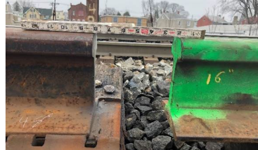
Figure 5 Example of Required Expansion Gap
