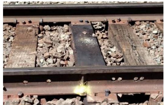
Figure 2 Field Weld Adjacent Tie
