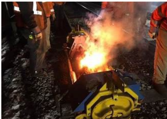
Figure 9 Closure welding with Rail Puller
