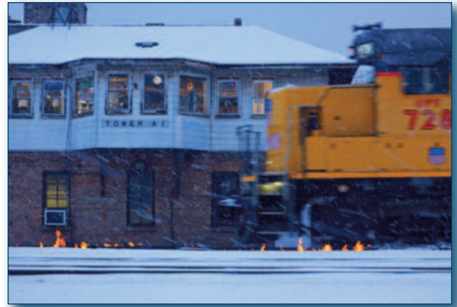
Three miles northwest of Chicago Union Station, Tower A-2, constructed in 1901, controls the movement of over 350 Amtrak, Metra and freight trains each weekday with a switching system that was installed in 1932. The open flames are used to keep switches free from ice because the tracks are not equipped with switch heaters.
