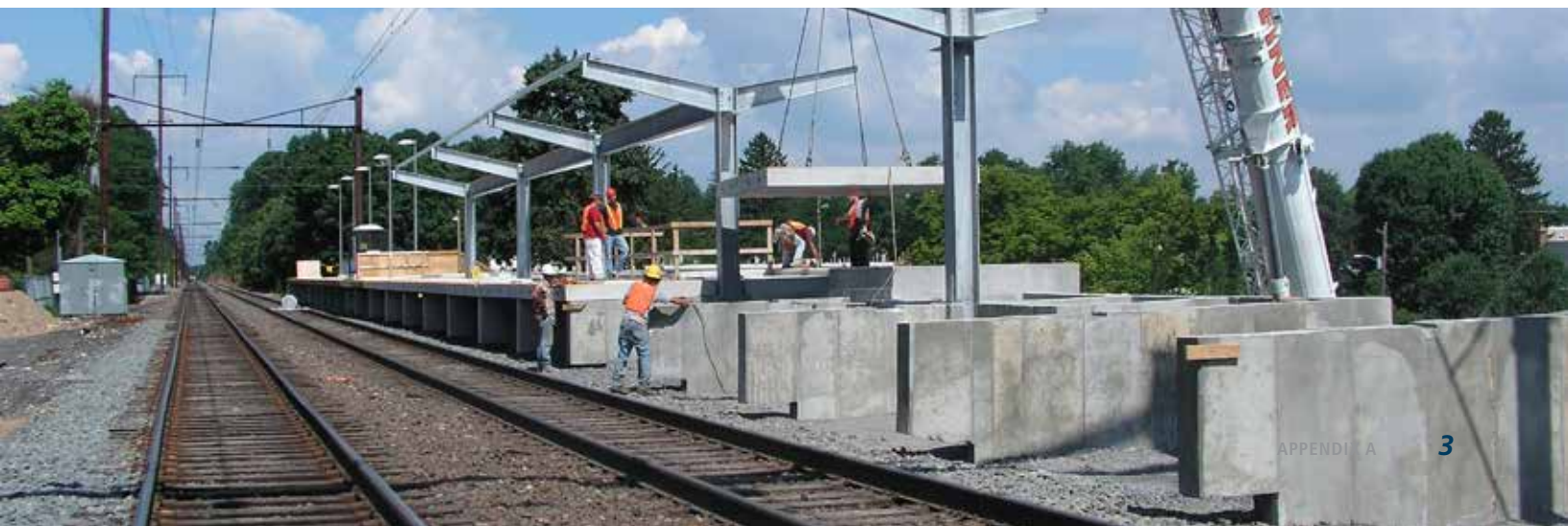
Below: Construction of ADA compliant platform at Elizabethtown, PA in 2010.
