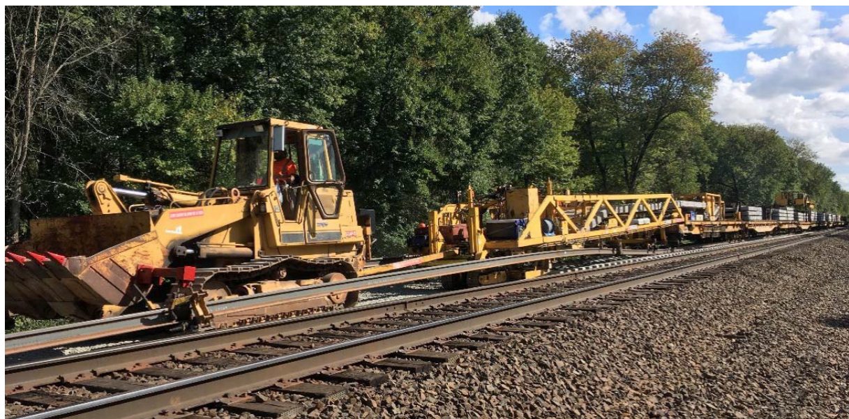
Track Laying Machine installing new second track.
