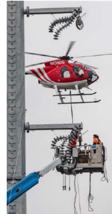
This photo was used last year. A helicopter strings rope during a power transmission pole wire installation in Newark, NJ. Photo by Amtrak/Marc Glucksman/River Rail Photo.
