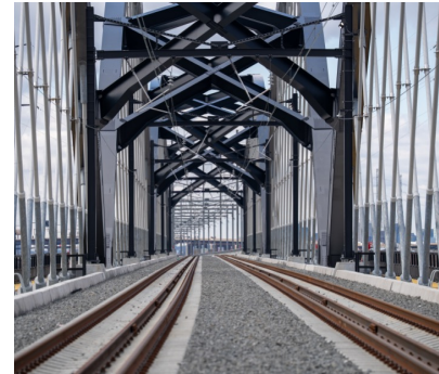
Portal North Bridge (Kearny, NJ)
