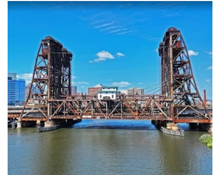
Dock Bridge (Newark, NJ)
