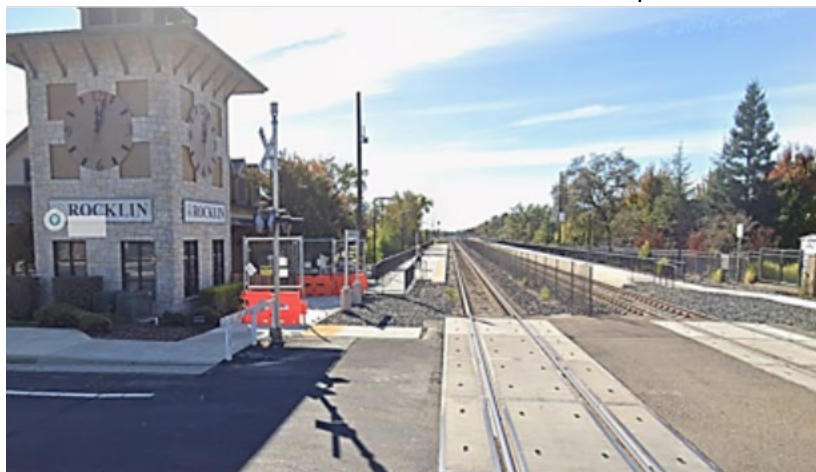
Figure 4 A glimpse of Rocklin Station, CA, with two new 512-foot platforms, lighting along the full length of the platform.
