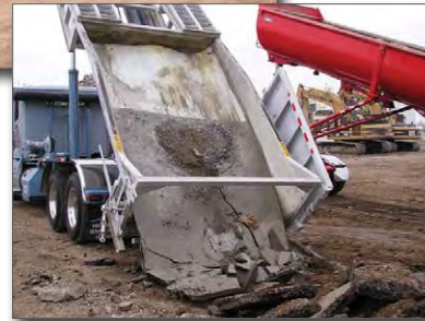
Figure 15. Delivering hardened Concrete to a recycler
