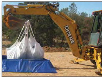
Figure 12. Extracting the concrete solids or gelled washwater
