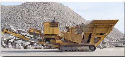
Figure 6. Crushed concrete stockpile and crusher
