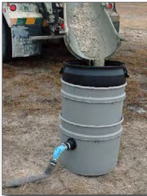
Figure 3. Concrete washout filter
