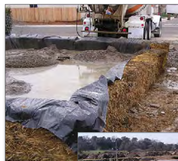
Figure 9. Hay bale and plastic washout pit
