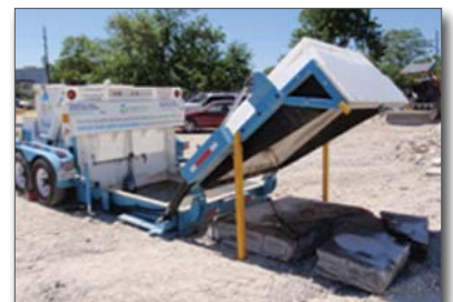
Figure 17. Delivering hardened concrete to a recycler
