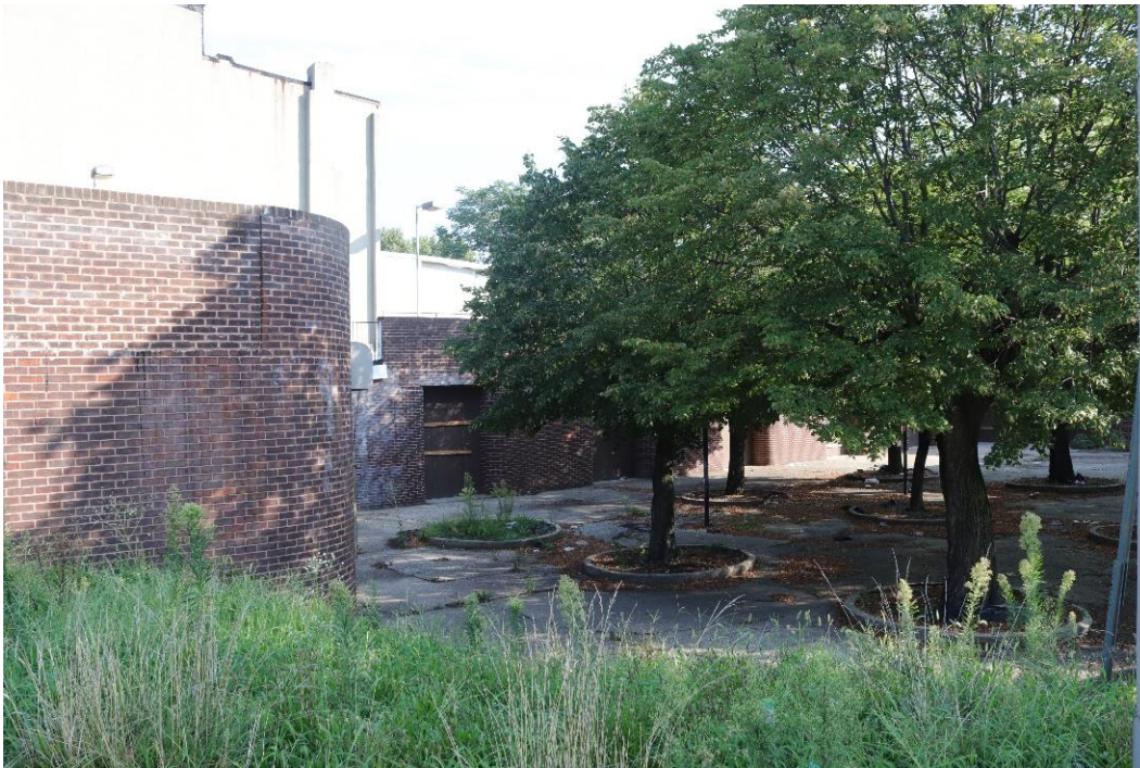
Photo 5: Southeast Elevation Facing the Courtyard, Looking Northwest
