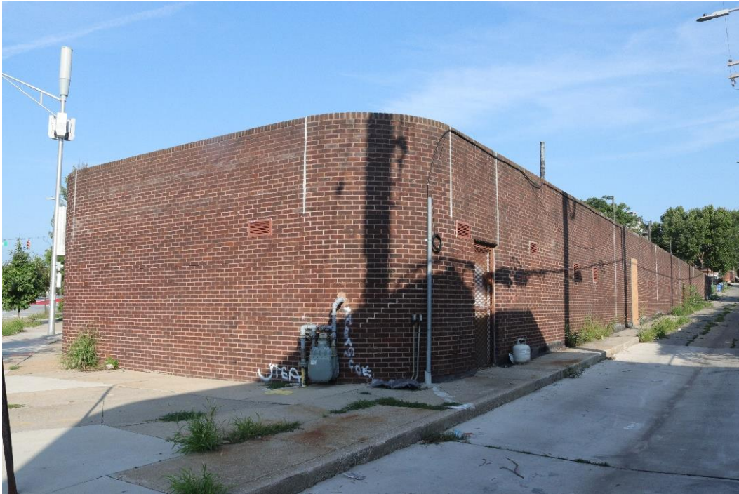
Photo 10: Southeast and Northeast Elevations, Looking Northwest
