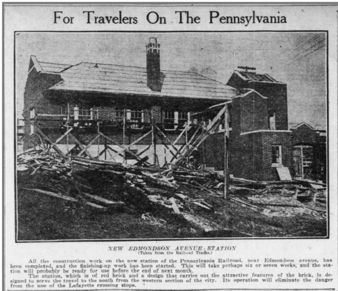
Figure 5. Photograph of the rear of the station during construction, looking northwest from the PRR tracks. "For Travelers on the Pennsylvania, New Edmondson Avenue Station," The Sun , 12 January 1917, https://www.newspapers.com , accessed 4 June 2019.
