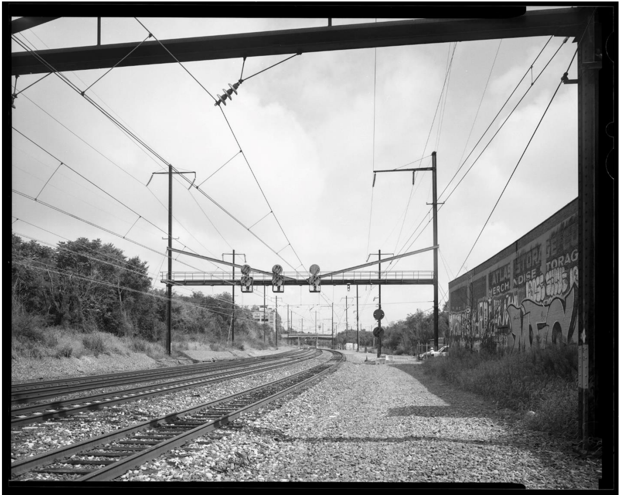
Figure 4. View of the Baltimore & Potomac Railroad corridor with the 1946 Atlas Storage Company Warehouse in the right foreground. Note “Atlas Storage Co. Merchandise Storage” painted on the wall above the graffiti. Rob Tucher, 2019, HAER No. MD-202-9.
