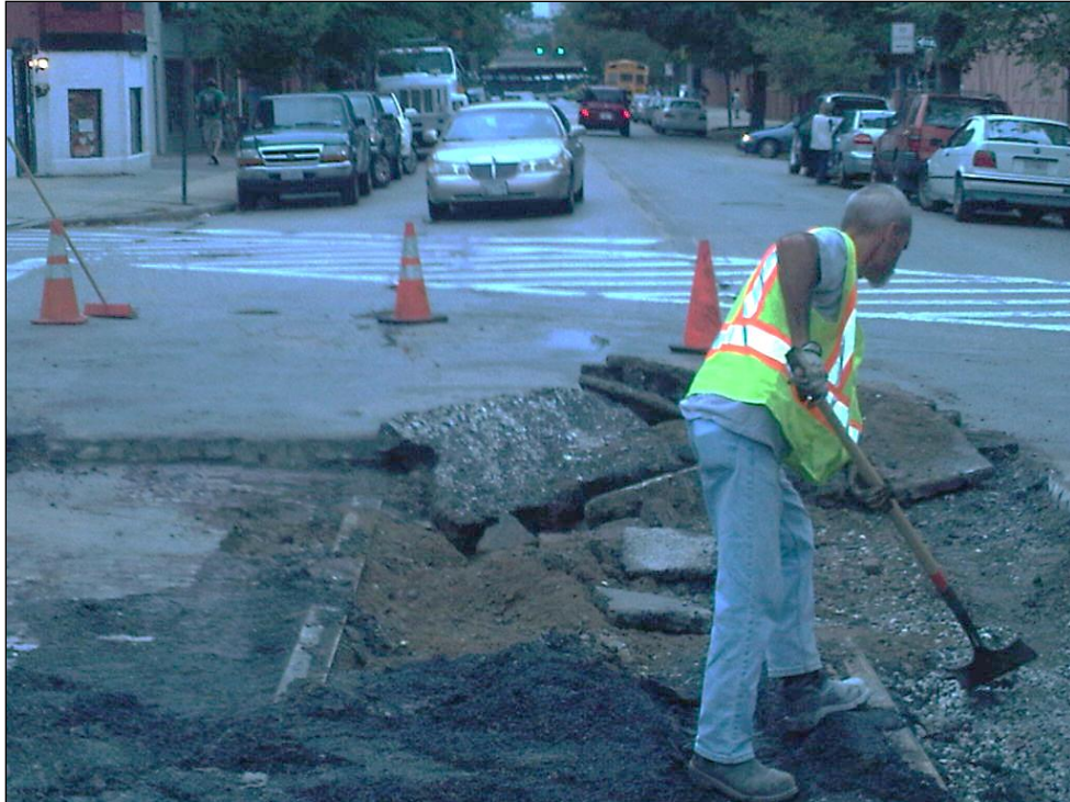
Figure 6: Intact Streetcar/Trolley Tracks, as exposed in street.
