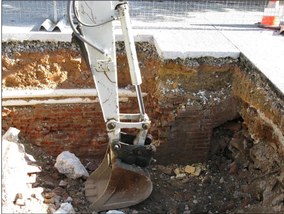
Figure 9: Intact Brick Foundation, as exposed in excavation.
