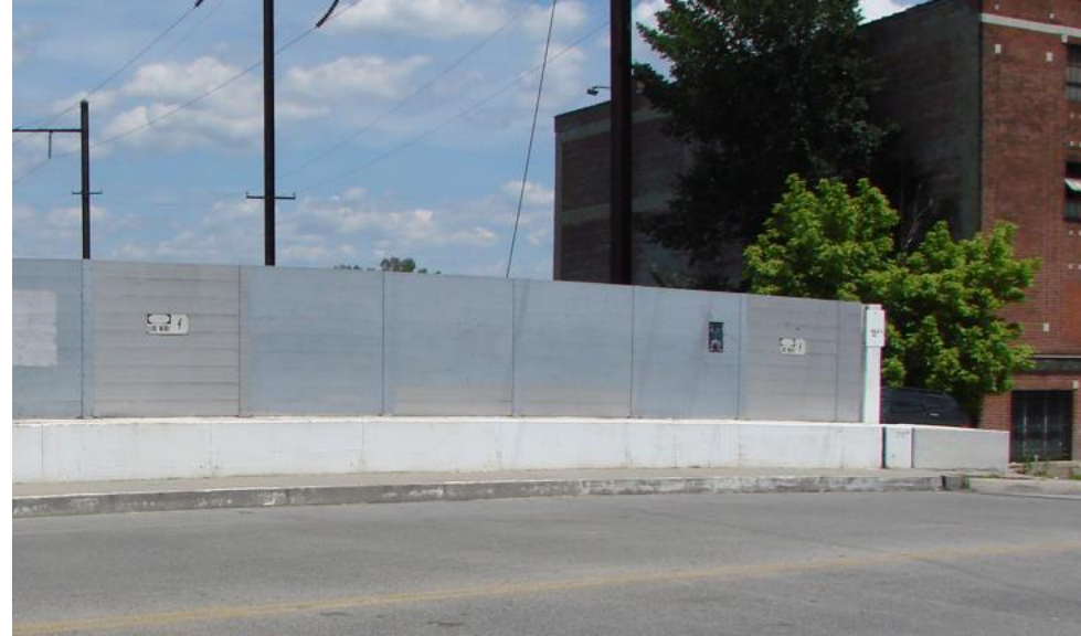
Traditional Barrier over Railroad (Existing Edmondson Bridge)
