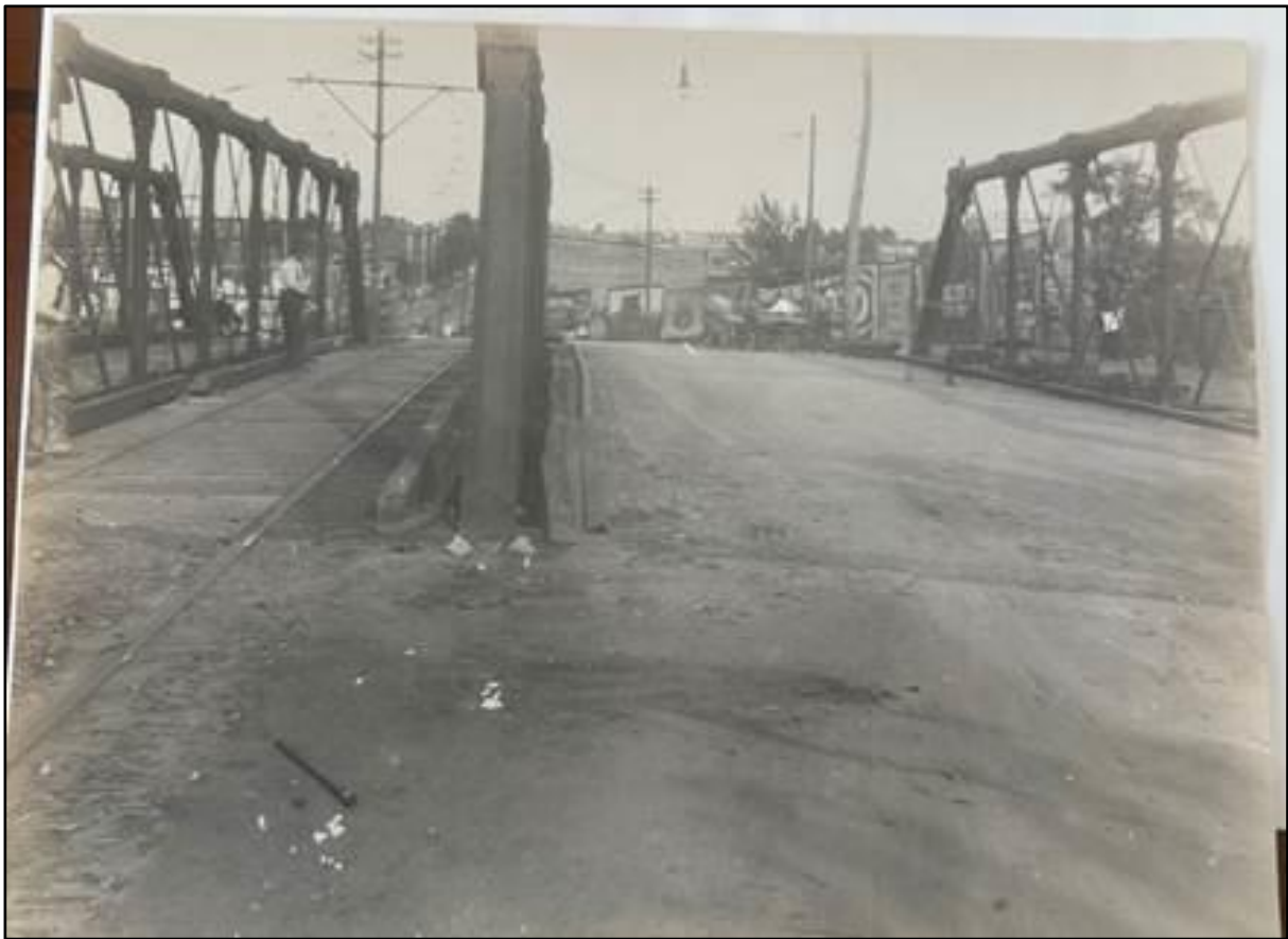
Figure 5: 1913 Photograph of the Edmondson Avenue Truss Bridge, on file at the Enoch Pratt Free Public Library.
