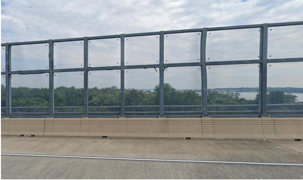
Clear Panel with angled or curved top (Woodrow Wilson Bridge)
