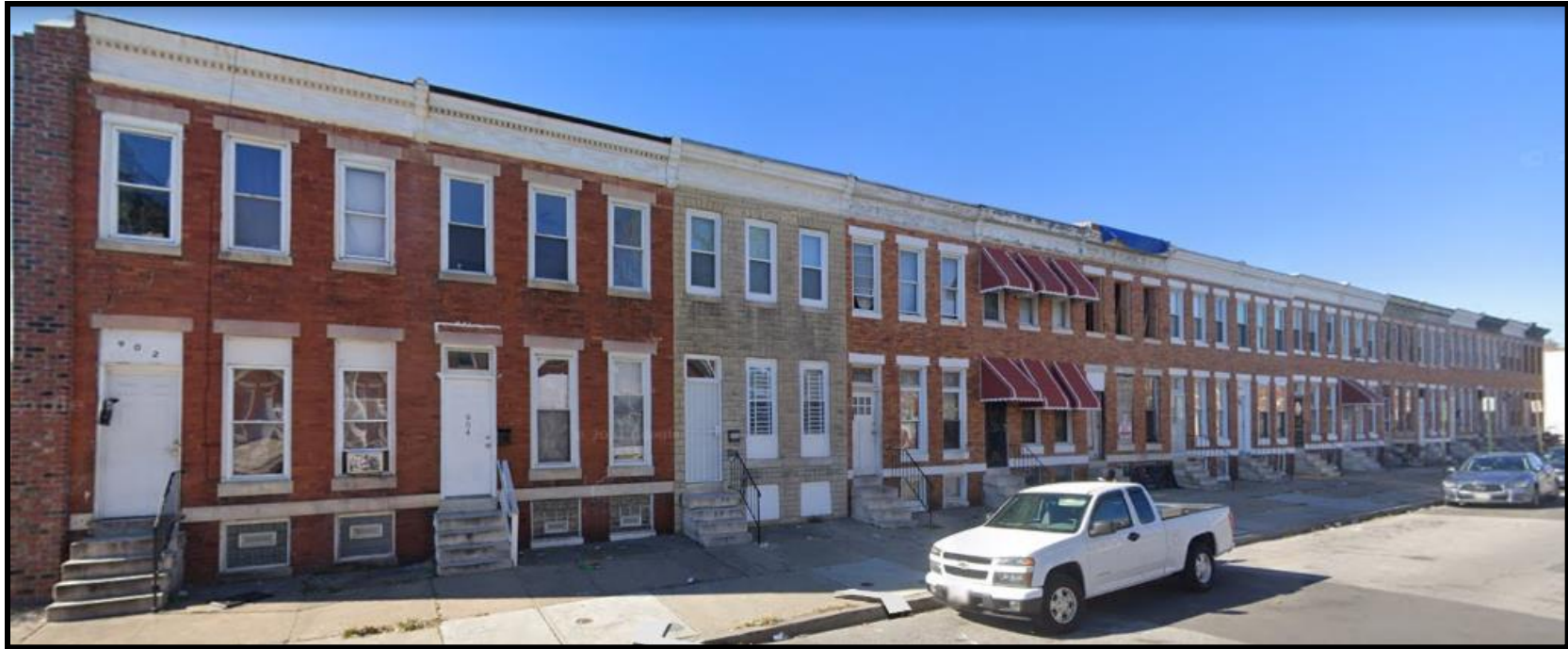
Above: View looking northwest at the 902-932 North Payson Street rowhouses (via Google Earth)
