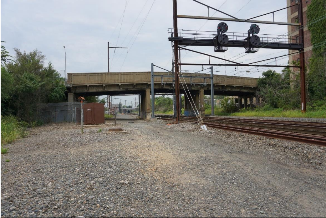
Figure 1: West Lafayette Avenue Bridge, view looking southwest. Photographer: Nancy Zerbe
