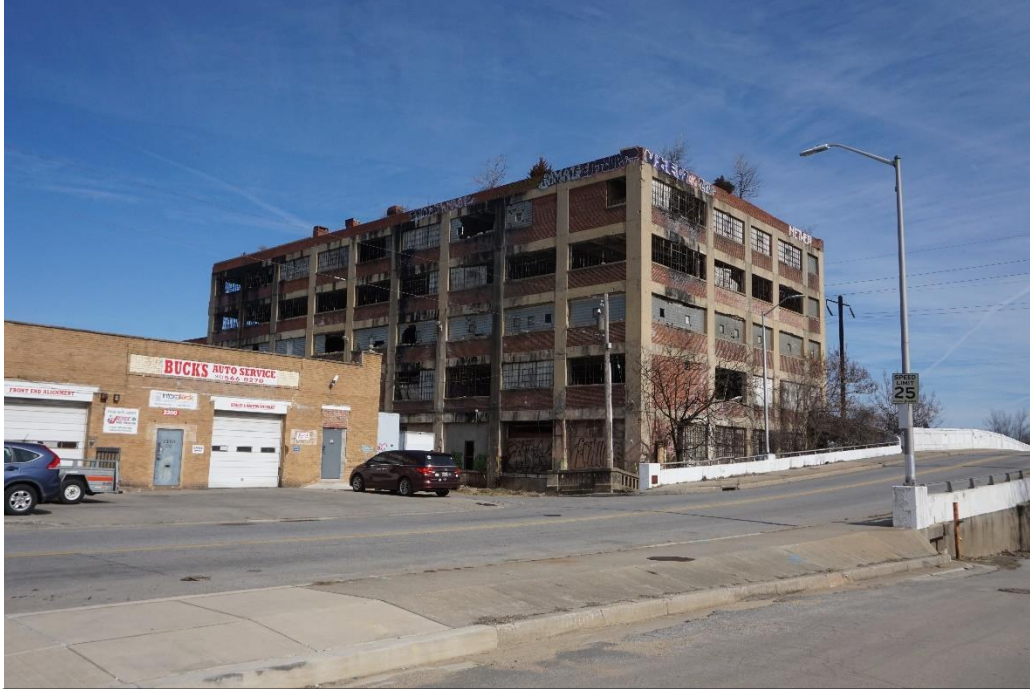
Figure 3: Western approach to the West Lafayette Avenue Bridge, five-story 2120 West Lafayette Avenue and one-story 2200 West Lafayette Avenue, view looking northeast. Photographer: Benny Louie.
