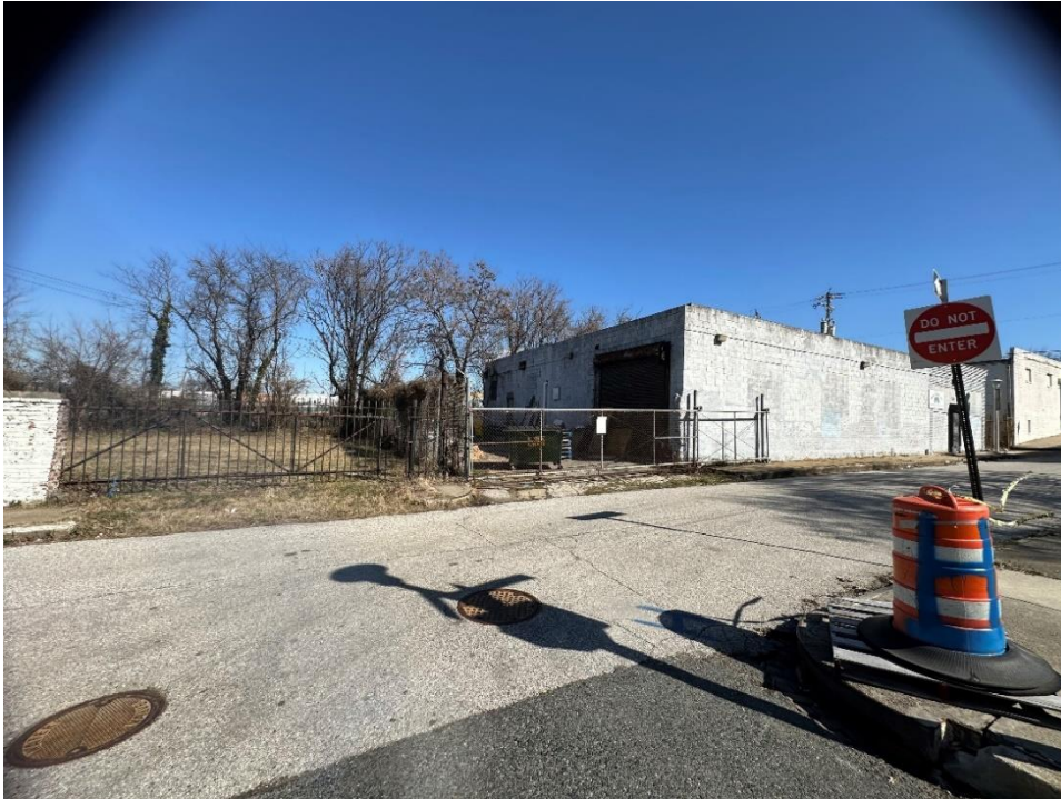
Figure 9: Industrial buildings at the intersection of Winchester Street and McKean Avenue, view looking northeast towards the rail line. Photographer: Nancy Zerbe.
