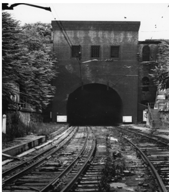
Pennsylvania Ave Station, tunnel approach
