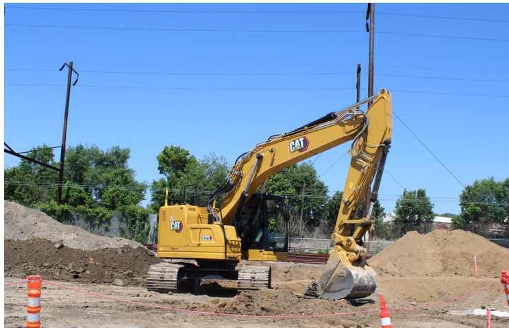
SOUTH PORTAL CONSTRUCTION SITE
