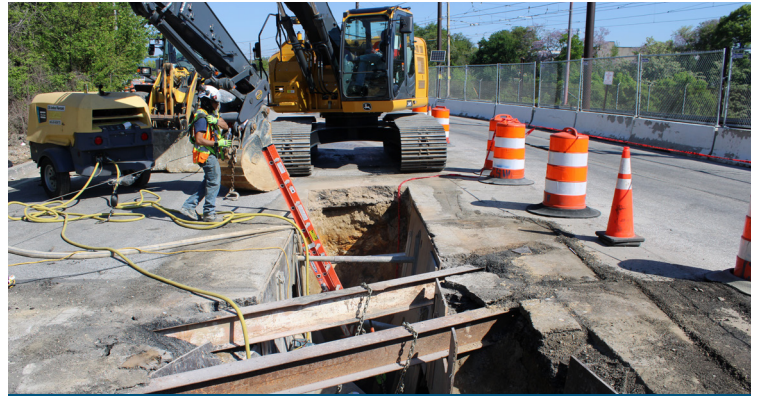
UTILITY RELOCATIONS ALONG MCMECHEN STREET
