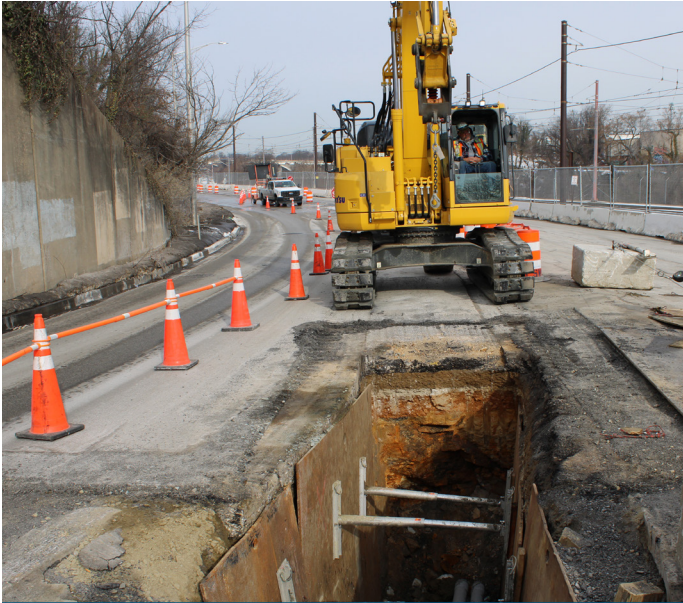
UTILITY INSTALLATIONS ON MCMECHEN STREET
