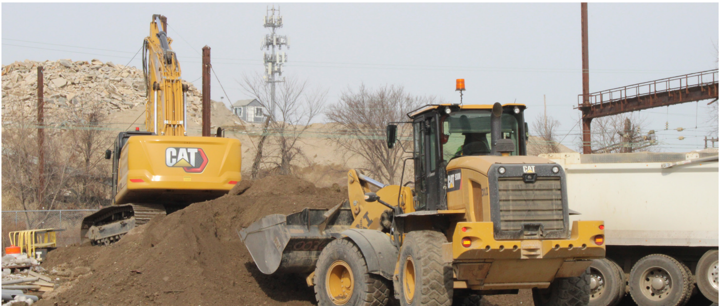
CONSTRUCTION SITE ON N PAYSON STREET
