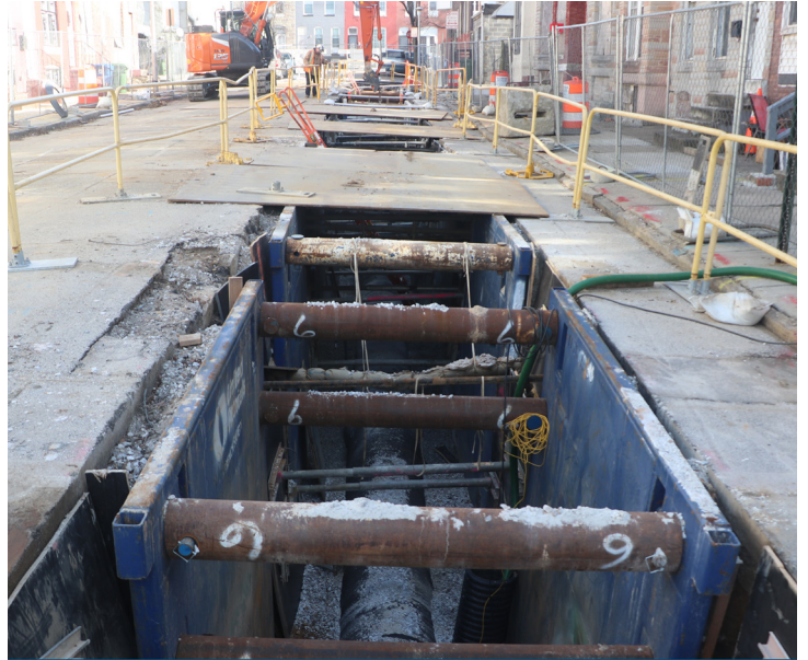
WATER LINE INSTALLATION ON RAYNER AVENUE
