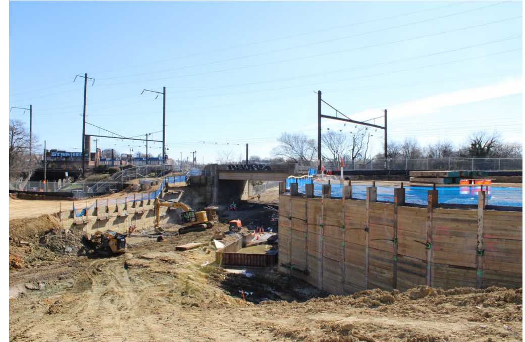
W Mulberry St Construction Activity
