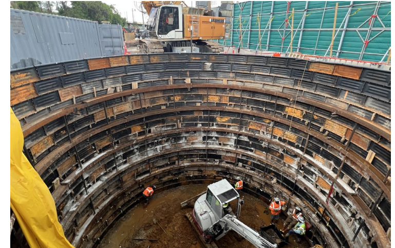
Liner plate and ring beams
