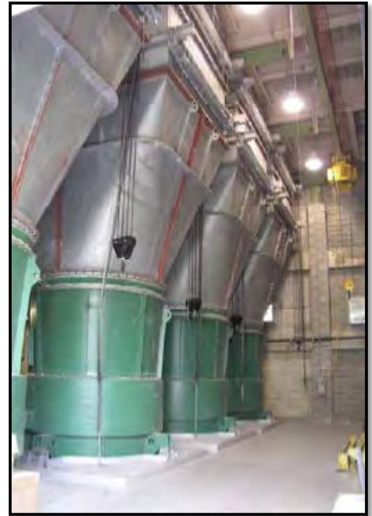
Figure 1: Tunnel Ventilation Fans at Amtrak Weehawken Shaft
