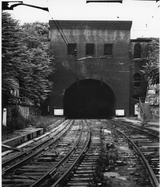
Pennsylvania Ave Station, tunnel approach
