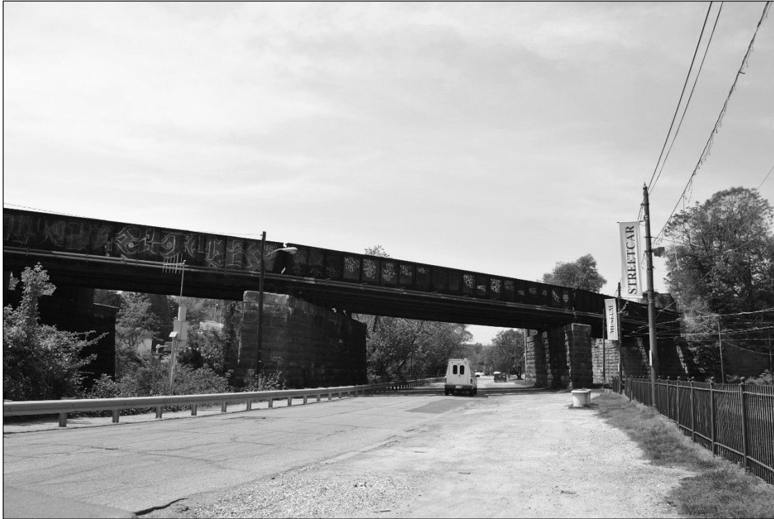
East Elevation of North End of B&O Baltimore Belt Line Bridge Over Jones Falls Valley, Showing the Three Deck-Plate Girders, Looking West.
