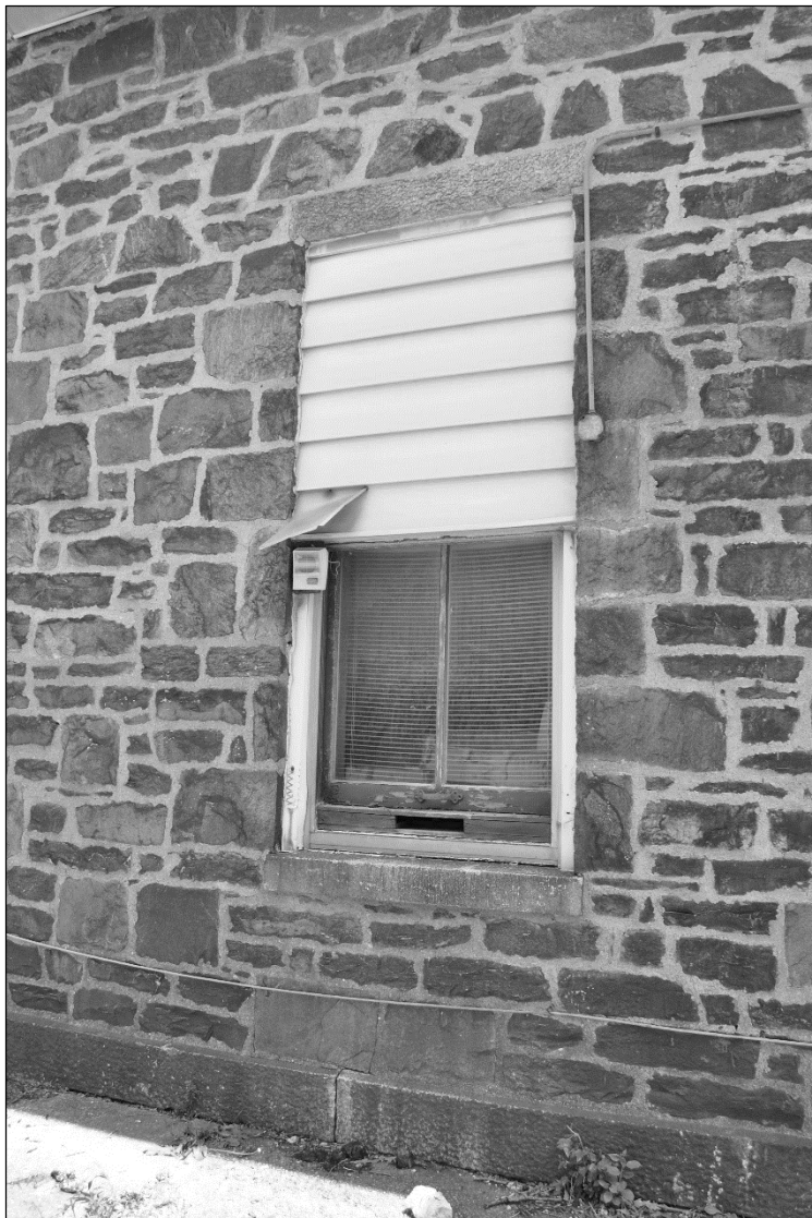
Detail of Partially Covered Wood Sash Window with Vertical Muntins on West Elevation, Looking Northeast.
