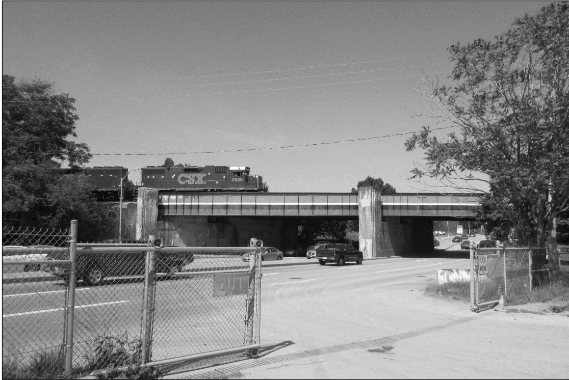
Double-Span, Steel Deck-Plate Girder Bridge with Concrete Abutments and Central Pier over Pulaski Highway/Route 40, Looking Northeast.
