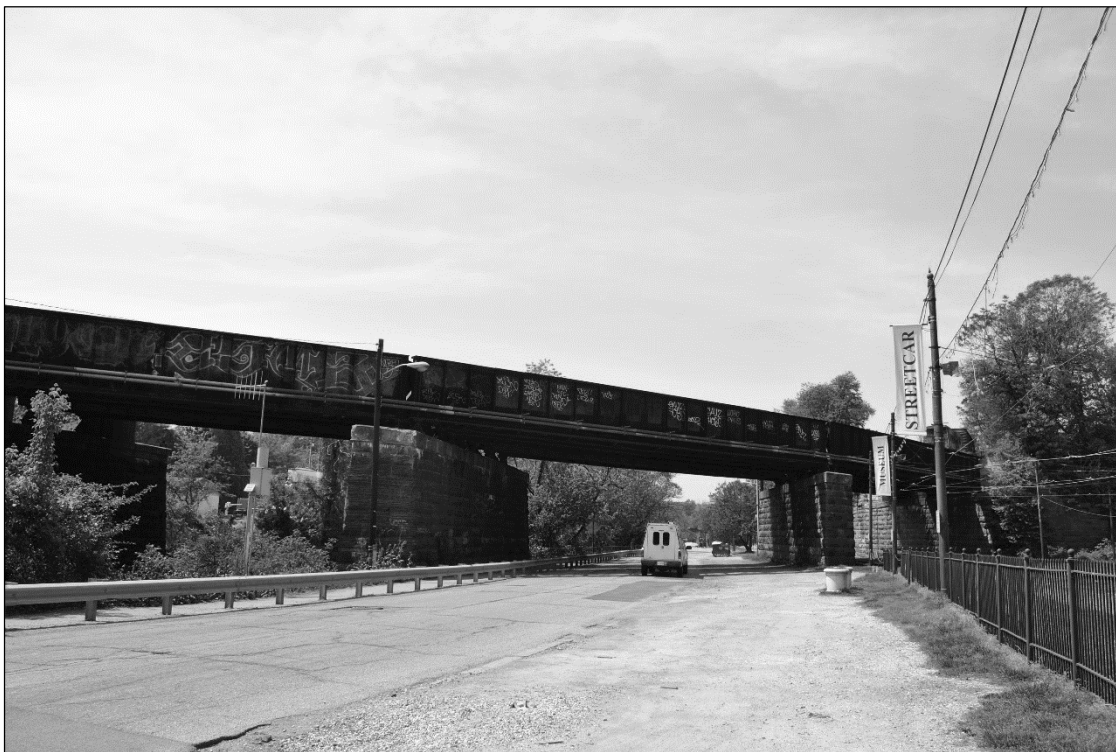
East Elevation of North End of Bridge, Showing the Three Deck-Plate Girders Over Jones Falls, Falls Road, and the Former Track ROW of the M&P Railroad, Looking West.
