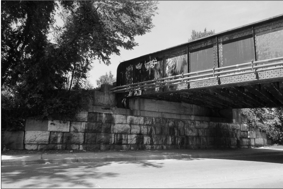
Single-Span, Through-Plate Girder Bridge over Saint Lo Drive, Showing Stepped Stone Abutment with Concrete Alterations and Repairs, Looking South.
