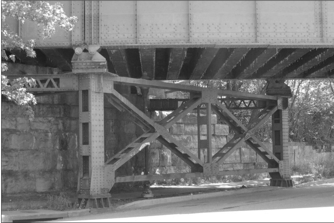
Detail of Steel Supports for Through-Plate Girder Bridge over Belair Road/Route 1, Looking South.
