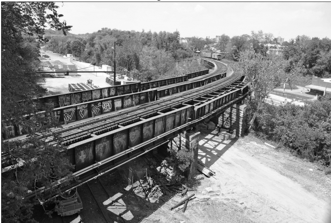
View of the B&O Baltimore Belt Line Bridge over Jones Falls Valley, Showing the Three Through-Plate Girders Over the Former Tracks of the PRR and Jones Falls, Looking North.
