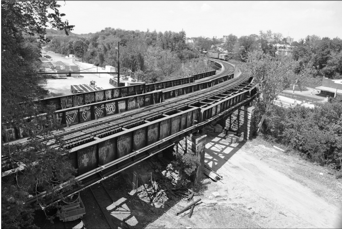
View of the B&O Baltimore Belt Line Bridge over Jones Falls Valley, Showing the Three Through-Plate Girders over the Former Alignment of the PRR and Jones Falls, Looking North.
