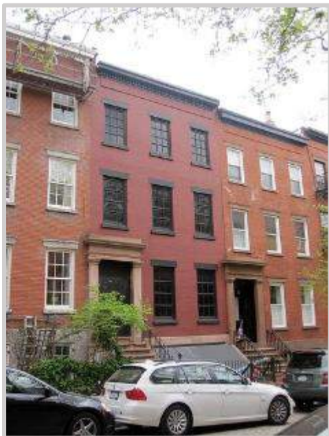
Image 1: Existing Ventilation Plant, 58 Joralemon Street, Brooklyn, NY
